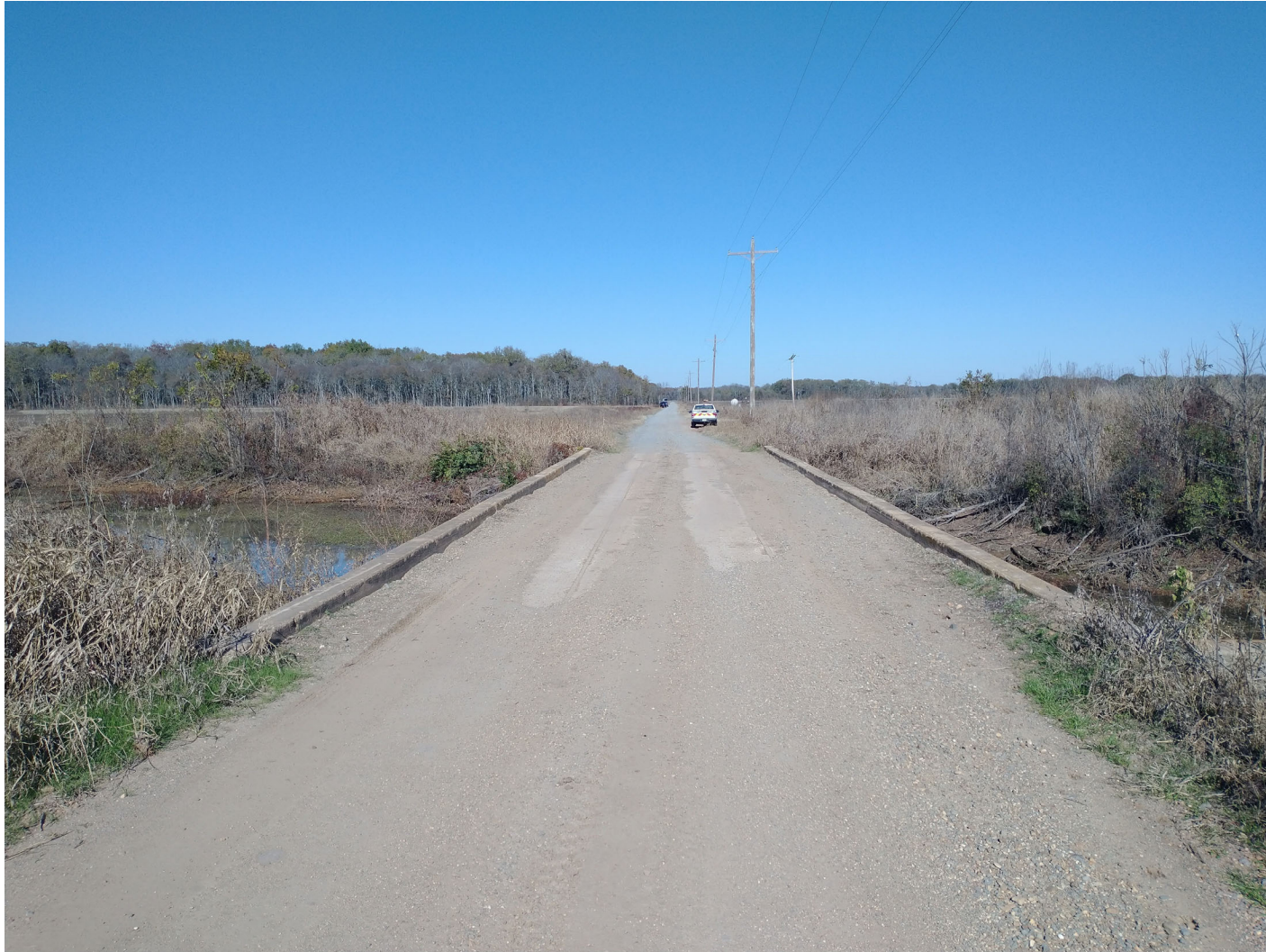
Looking North at Existing Bridge (November 2023)
