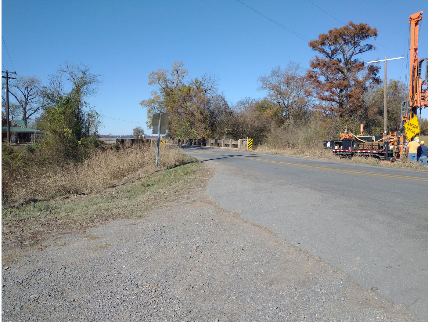
Looking West at Existing Bridge (November 2023)
