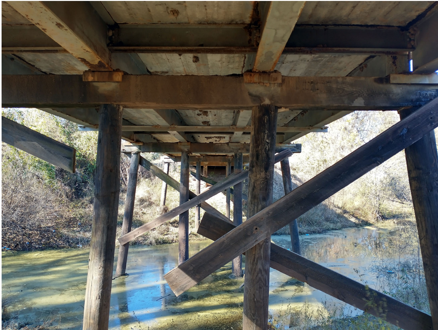
Looking East Under Existing Bridge (November 2023)
