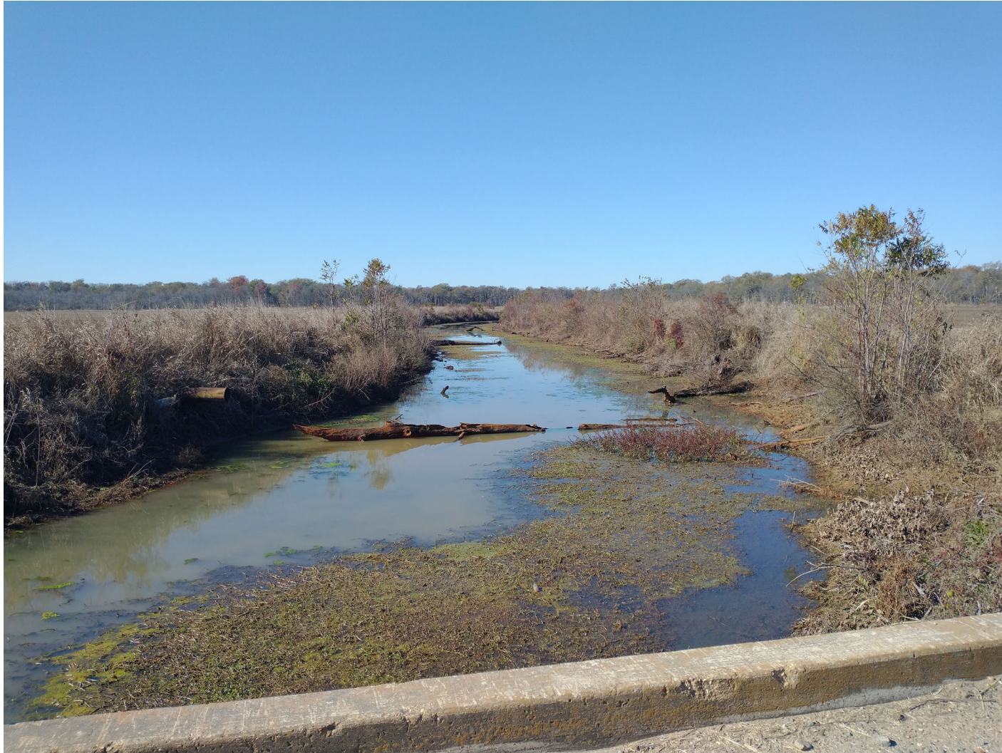
Looking West (Upstream) at Little Bayou Meto (November 2023)
