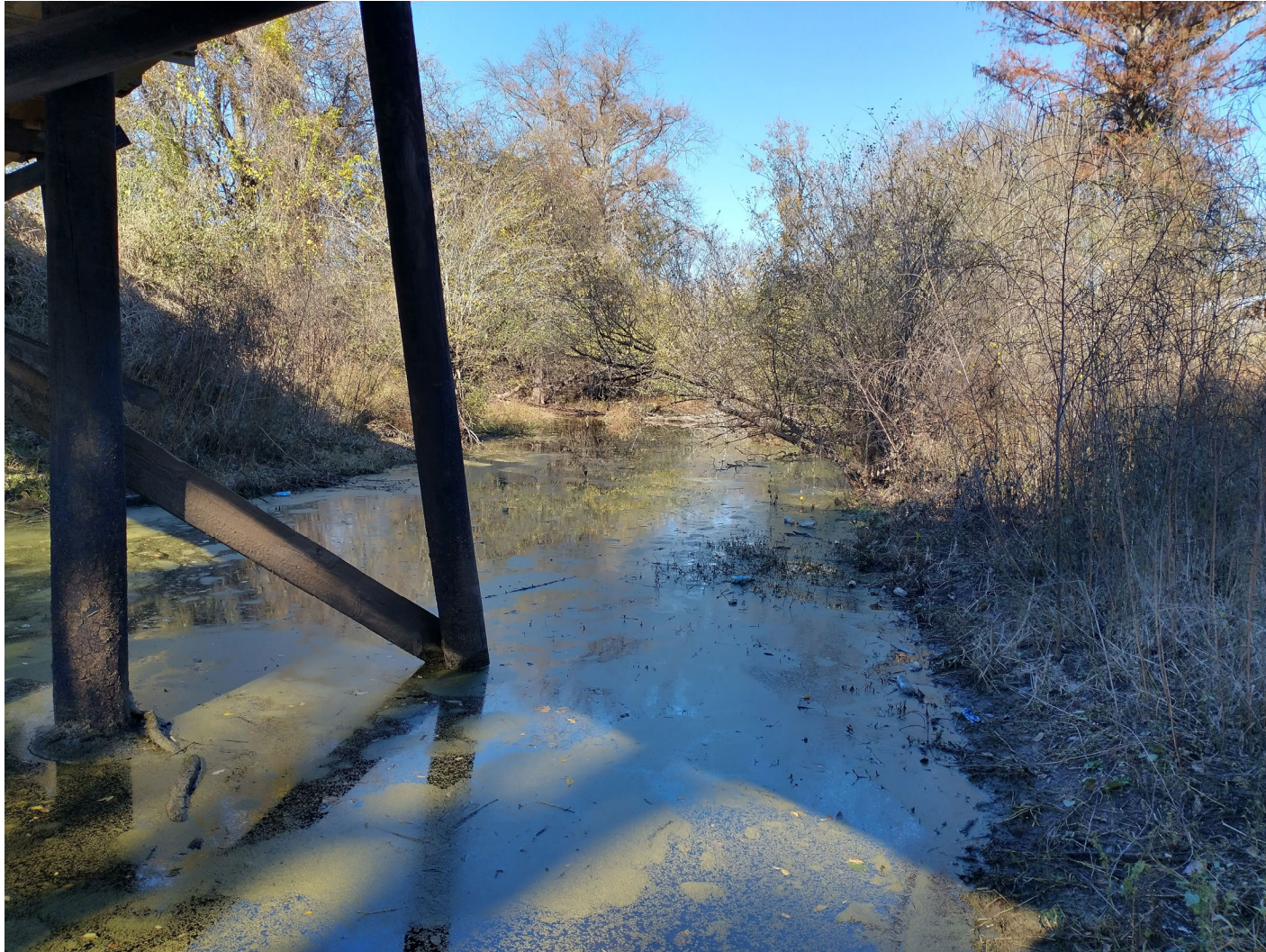
Looking Upstream at Little Bayou Meto Under Existing Bridge (November 2023)
