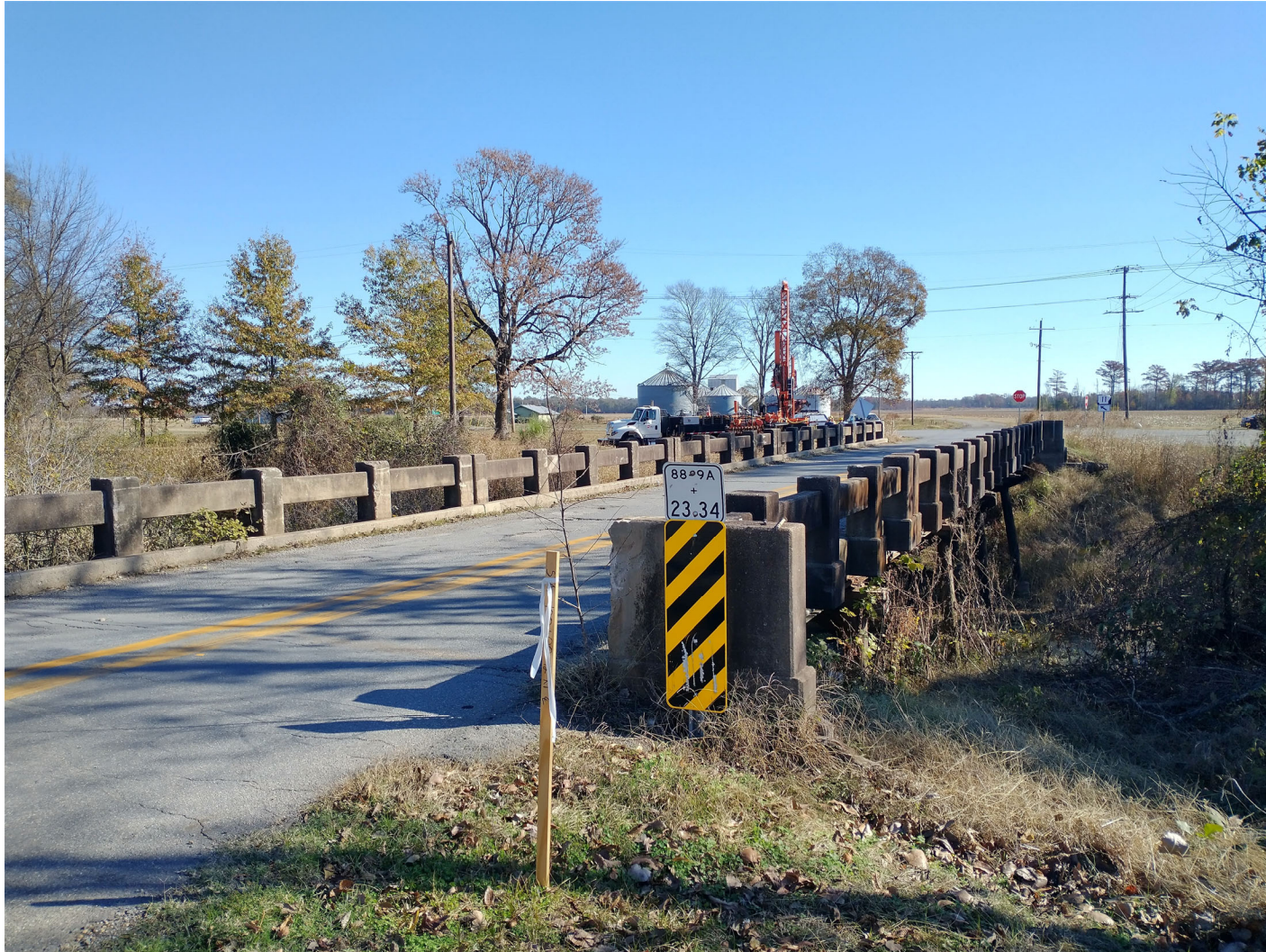
Looking East at Existing Bridge (November 2023)
