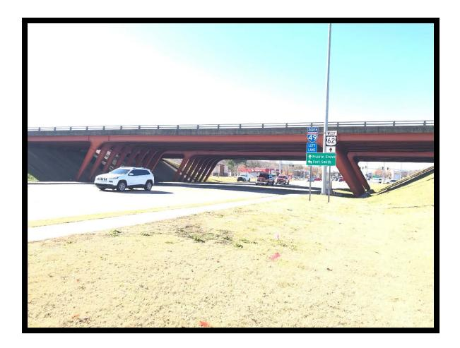
ARDOT Bridge Number 05074 is a steel continuous frame bridge carrying northbound Interstate 49 across Highway 62 in Washington County. McGeorge Contracting Company Inc. of Pine Bluff, Arkansas, constructed this bridge in 1971. Metal tube railings held by curved metal posts on low concrete parapets line the sides of the bridge. Its length totals 194 feet, with a clear roadway width of 43 feet, and it was built at an eight-degree skew.
