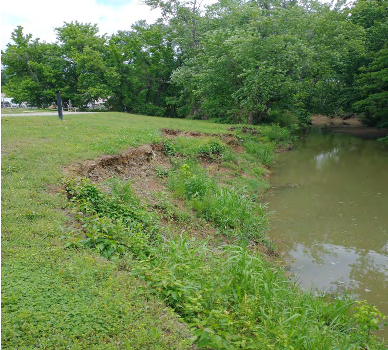
Looking north at scour on the northwest Heartsill Creek bank.
