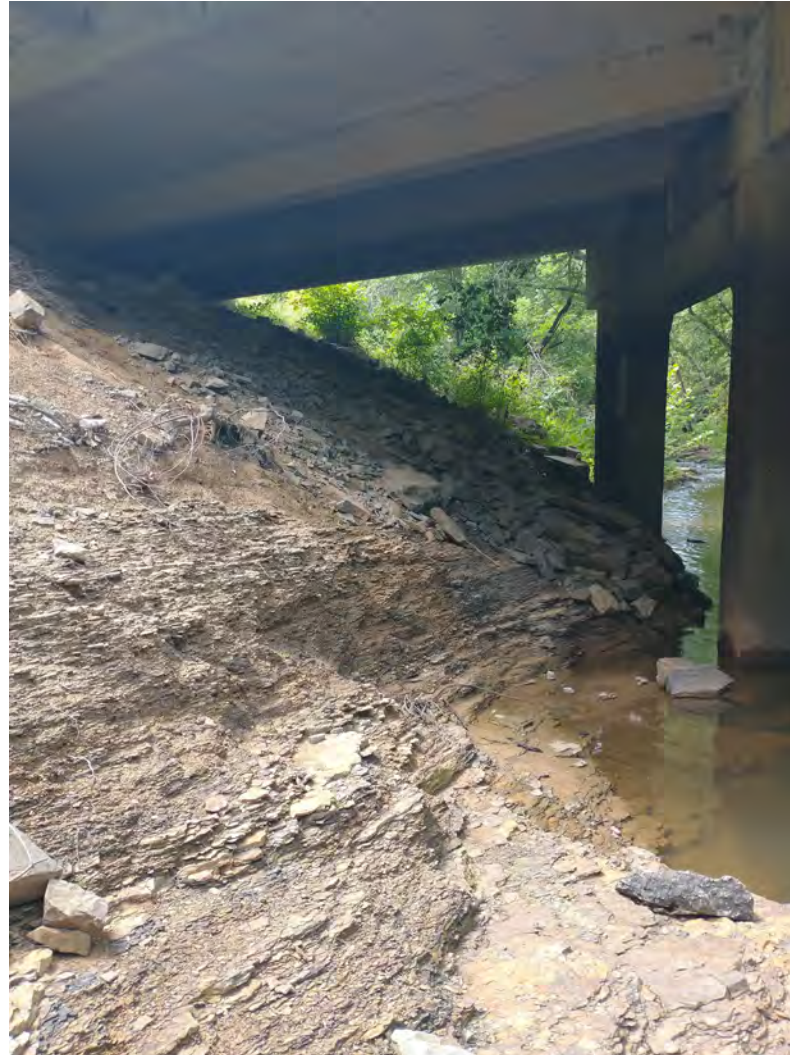
Looking south at shale exposed under southeast bridge end.
