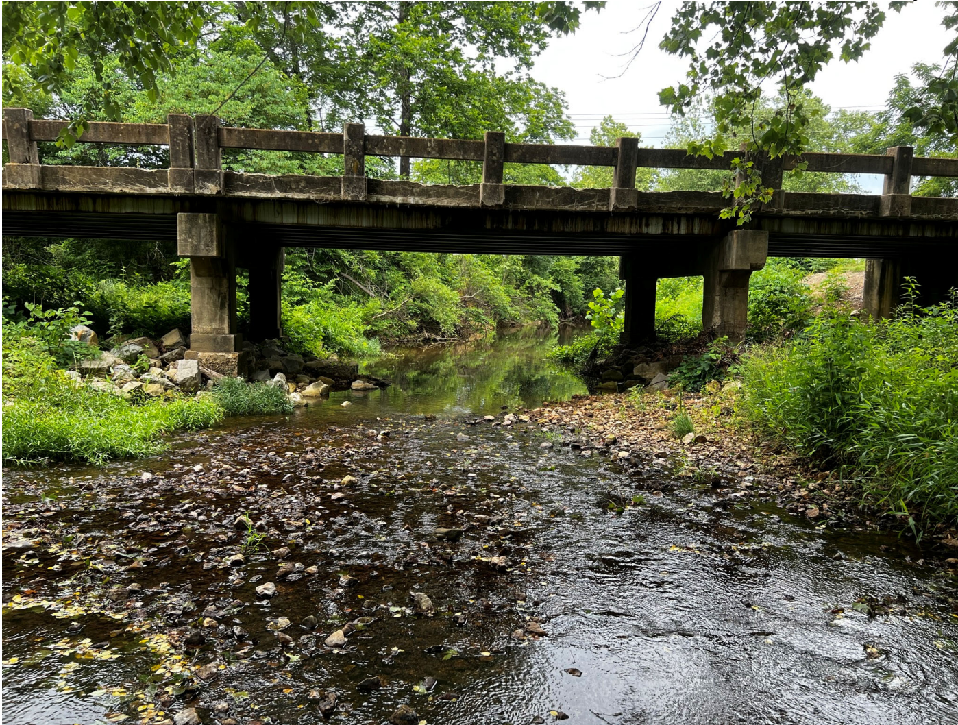
East side of existing bridge looking downstream (June 2023)
