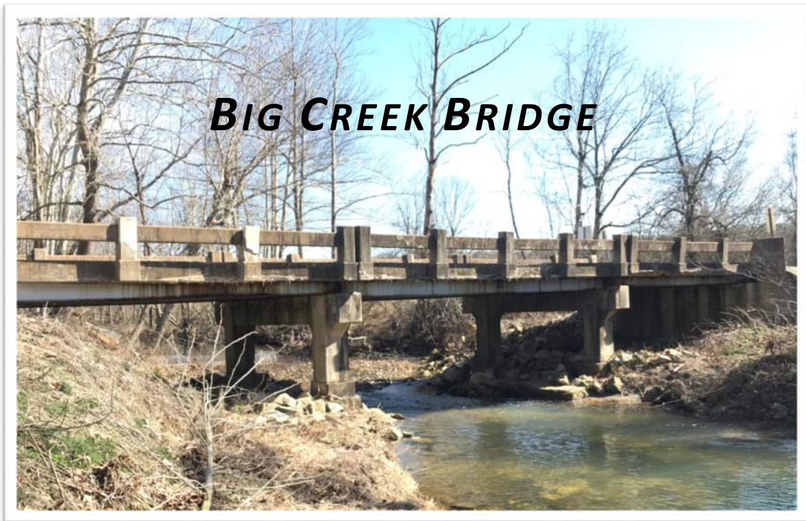
BRIDGE NUMBER M2381
