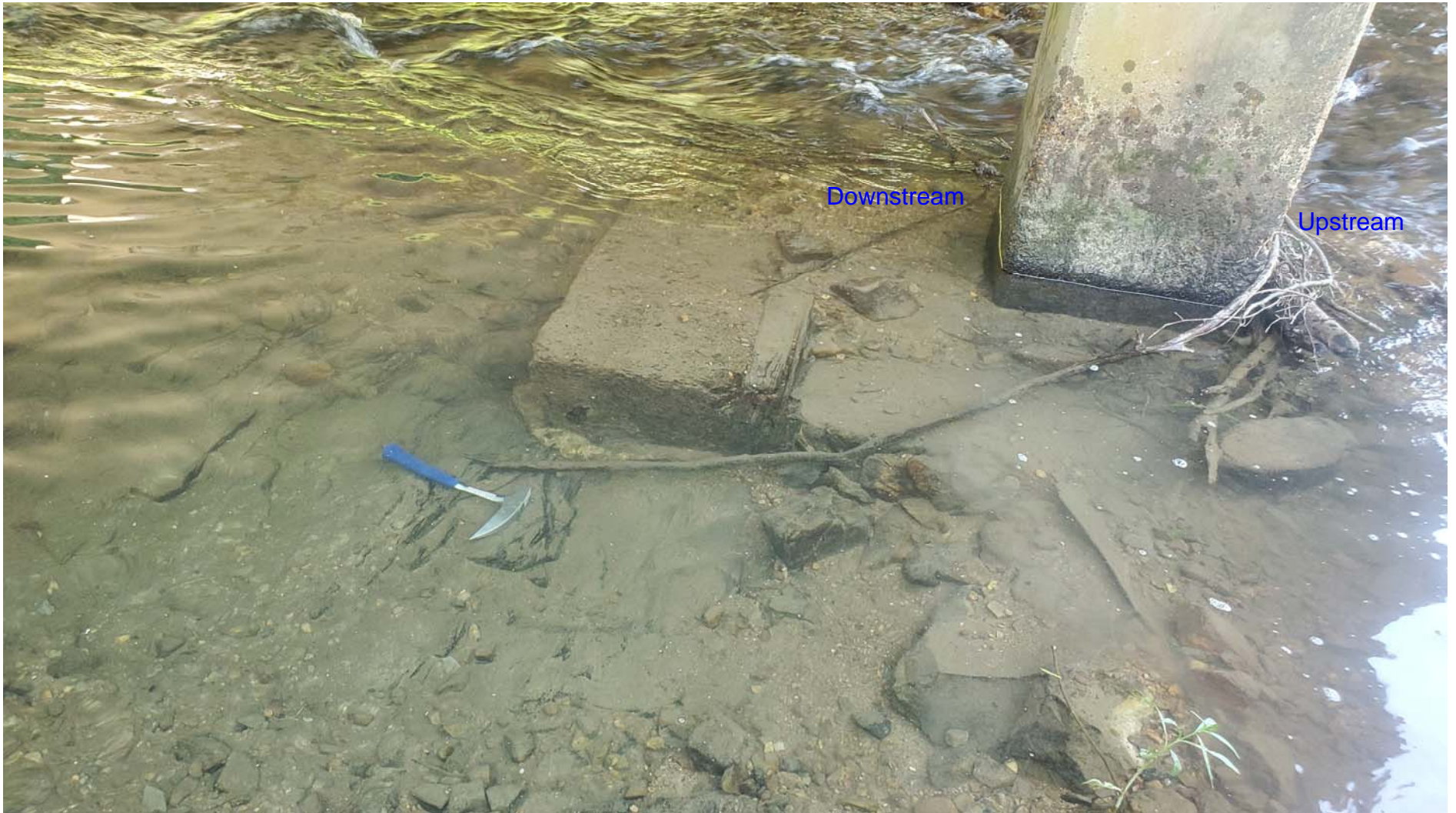
Scour around Footing and Exposed Shale (June 2021) Left Column – Bent 5
