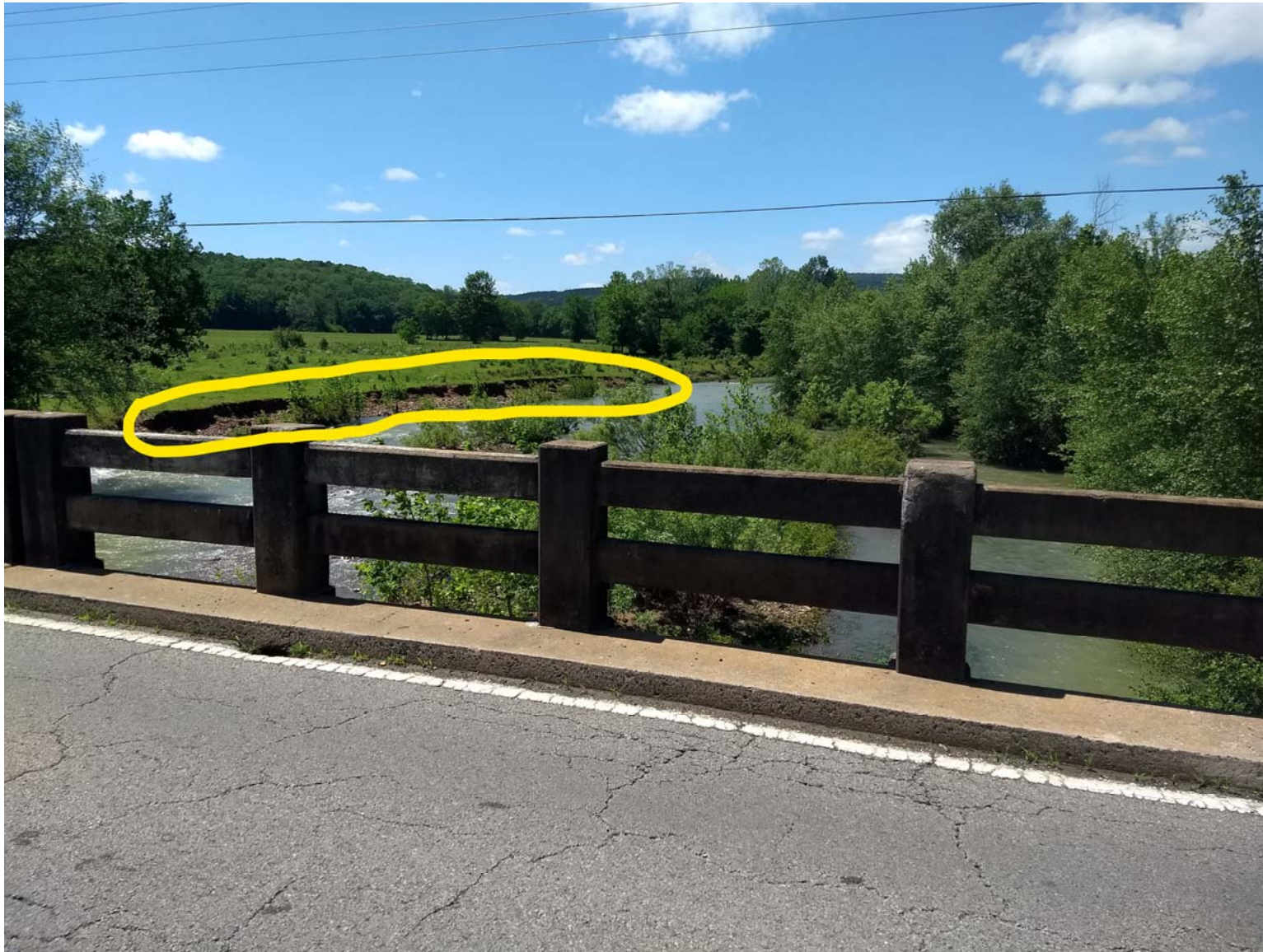
Minor Scour Observed on the Southwest Bank of the Creek (July 2021)
