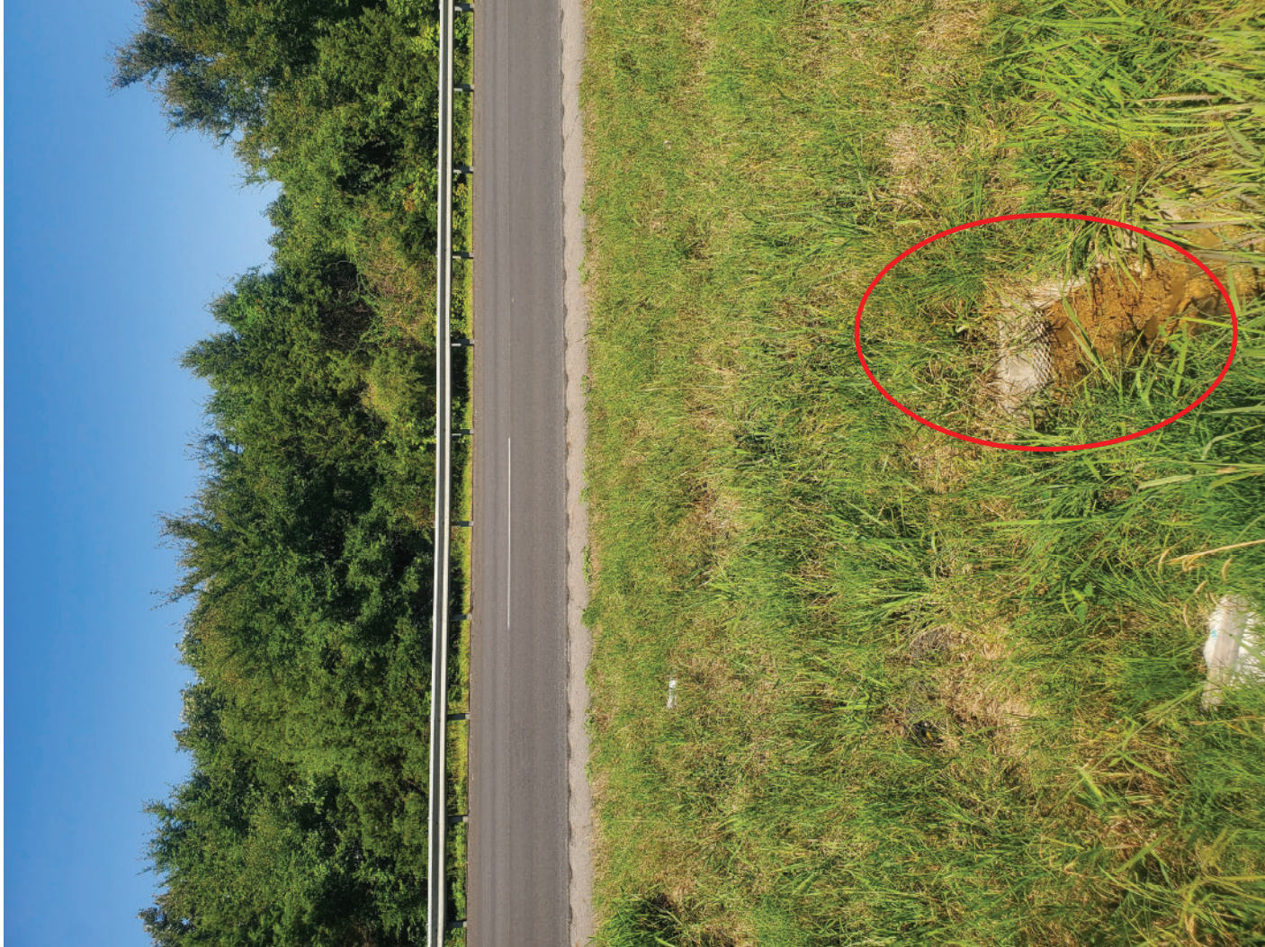
Clogged Pipe Underdrain in the Median (Slow Flowing to the East away from E Bound), Looking East (2022-08-18)
