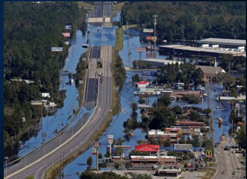
Source: North Carolina Department of Transportation
