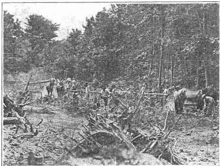
Two Views of Some Heavy Clearing and Grubbing Work on the Roads of Polk County
