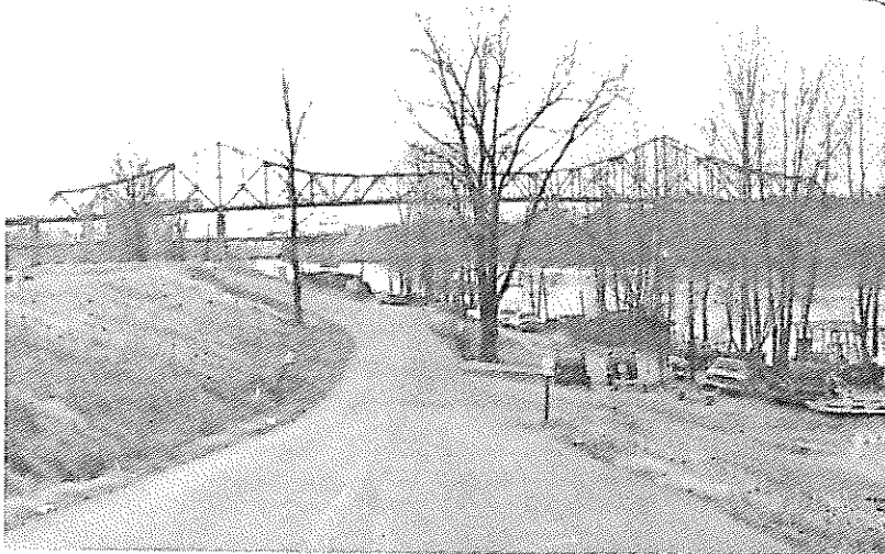
Bridge No. 1253, Type 310, steel through truss, double arch cantilever main span. U.S. Highway 79 over White River, Clarendon, Monroe County.
