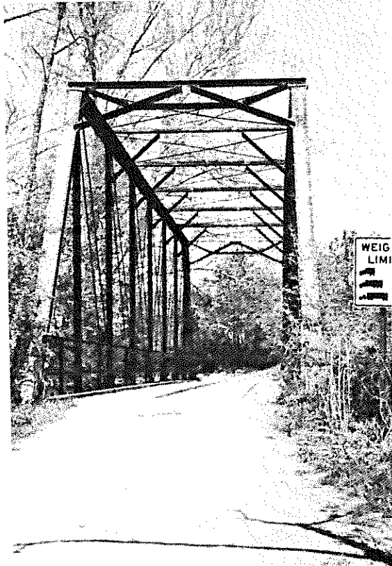
Bridge No. 10622, Type 310, Pratt through truss. Benton County Road 71 over Osage Creek.
