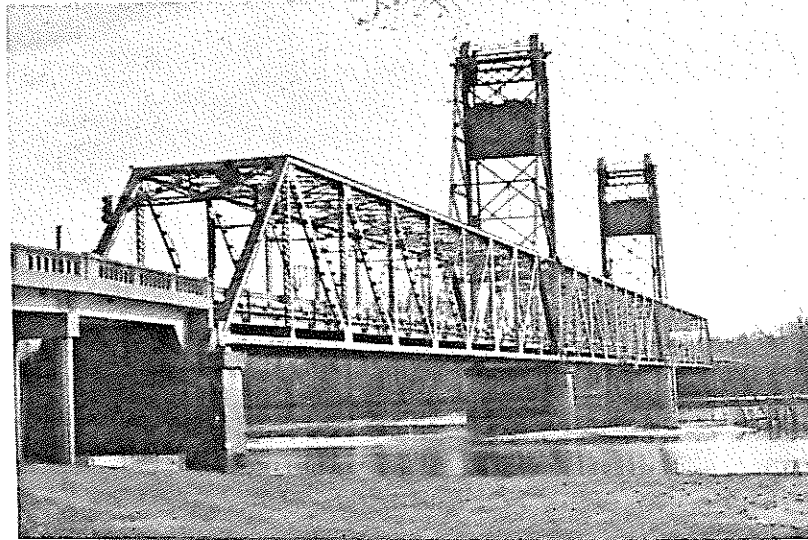
Bridge No. 1531, Type 310, steel through truss, life span. U.S. Highway 70 over White River, Prairie County.
