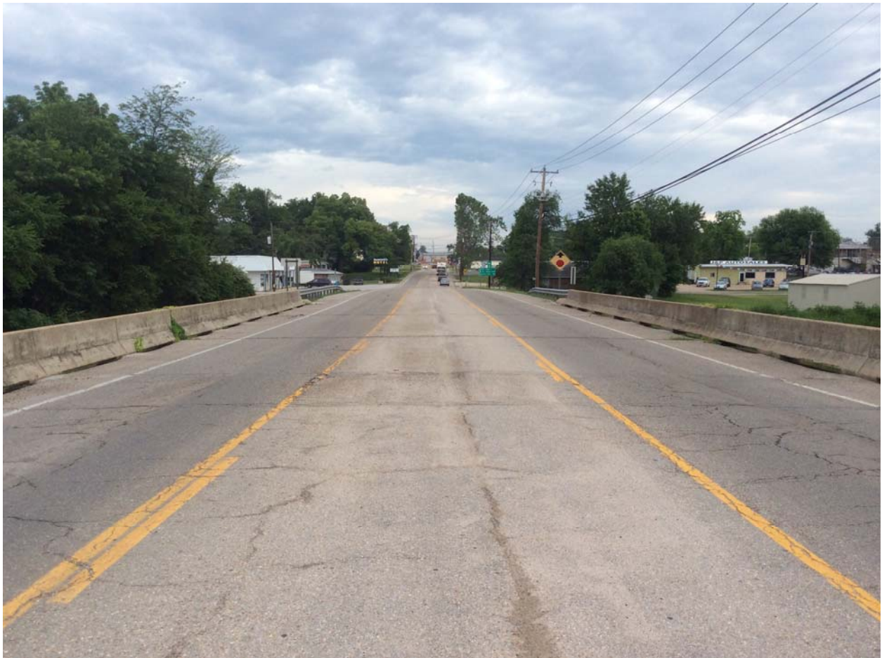
Note: 4.3" of ACHM overlay on bridge deck
