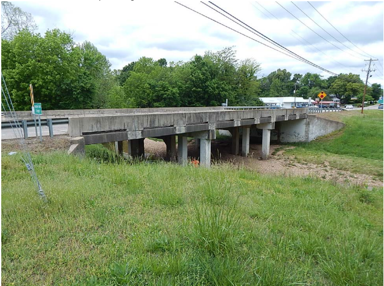
Note: 4.3" of ACHM overlay on bridge deck
