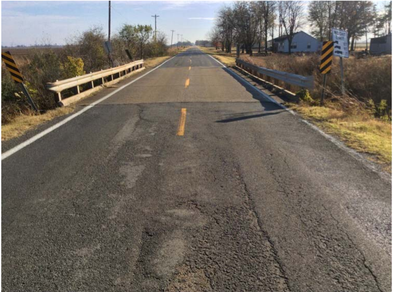
Note: Load postings and 4" of ACHM overlay on bridge deck.
