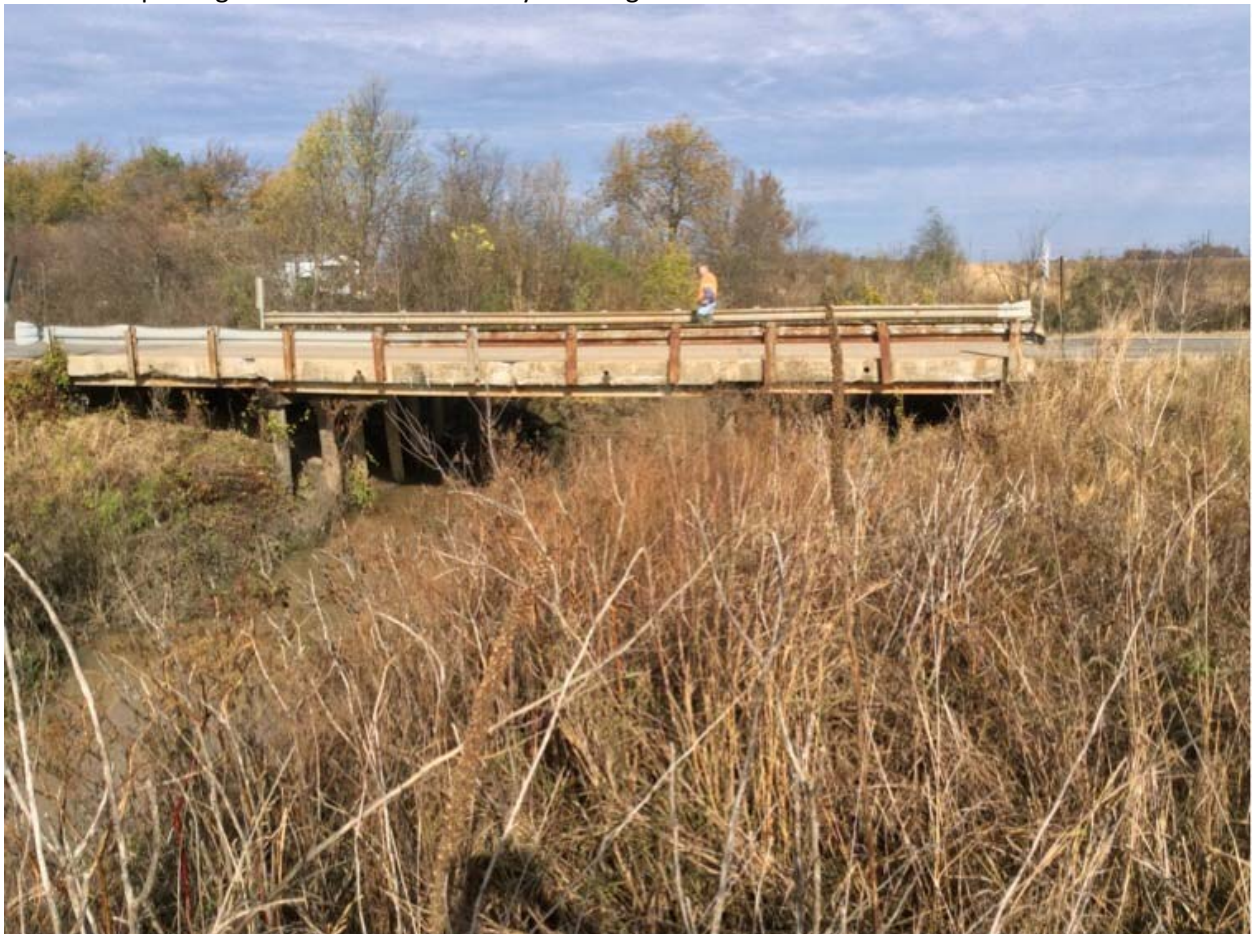
Note: Load postings and 4" of ACHM overlay on bridge deck.
