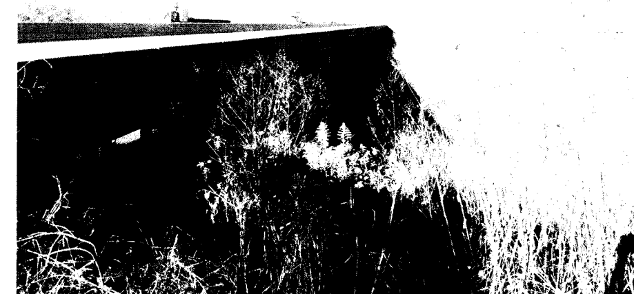
SITE NO. 6 - BRIDGE NO. A5447
