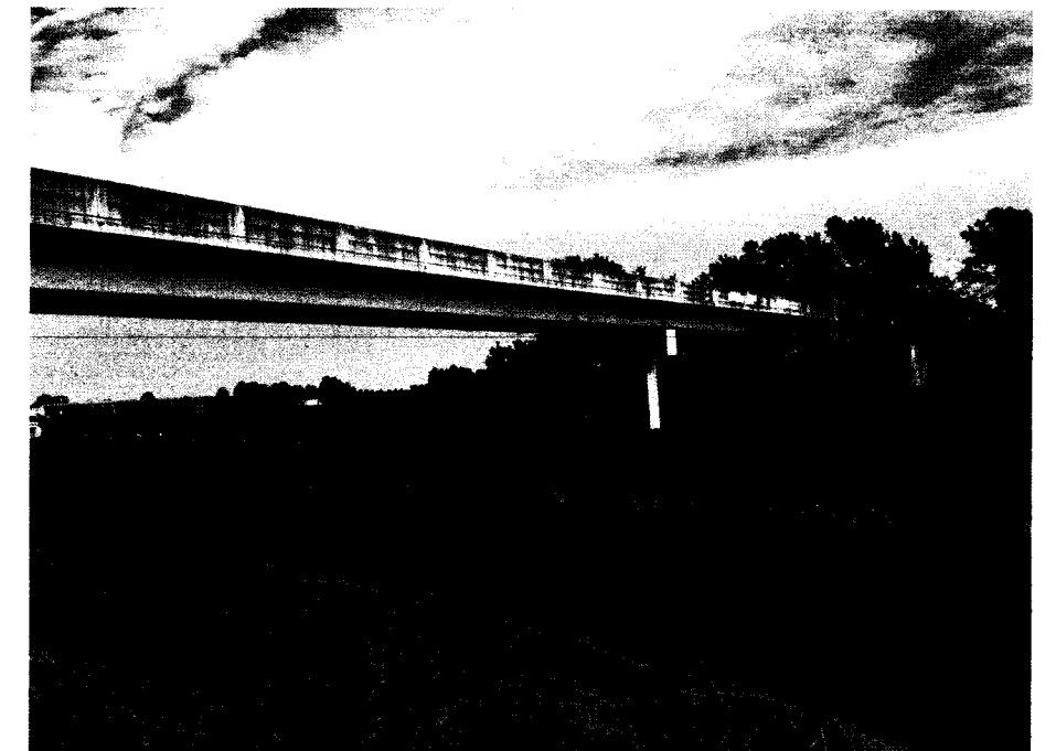
SITE NO. 12 - BRIDGE NO. 06040
