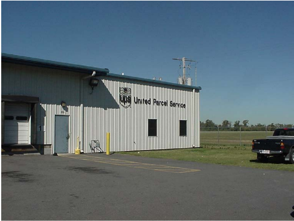
UPS Facility at Air Cargo Terminal
