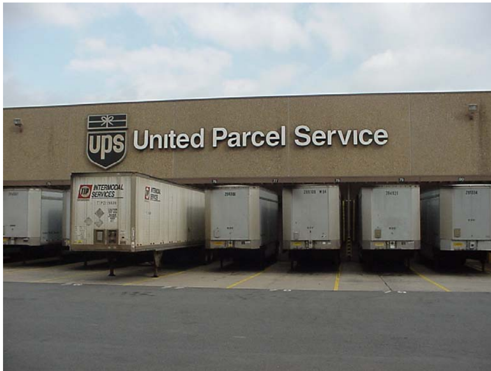
UPS Processing Center on Fourche Dam Pike
