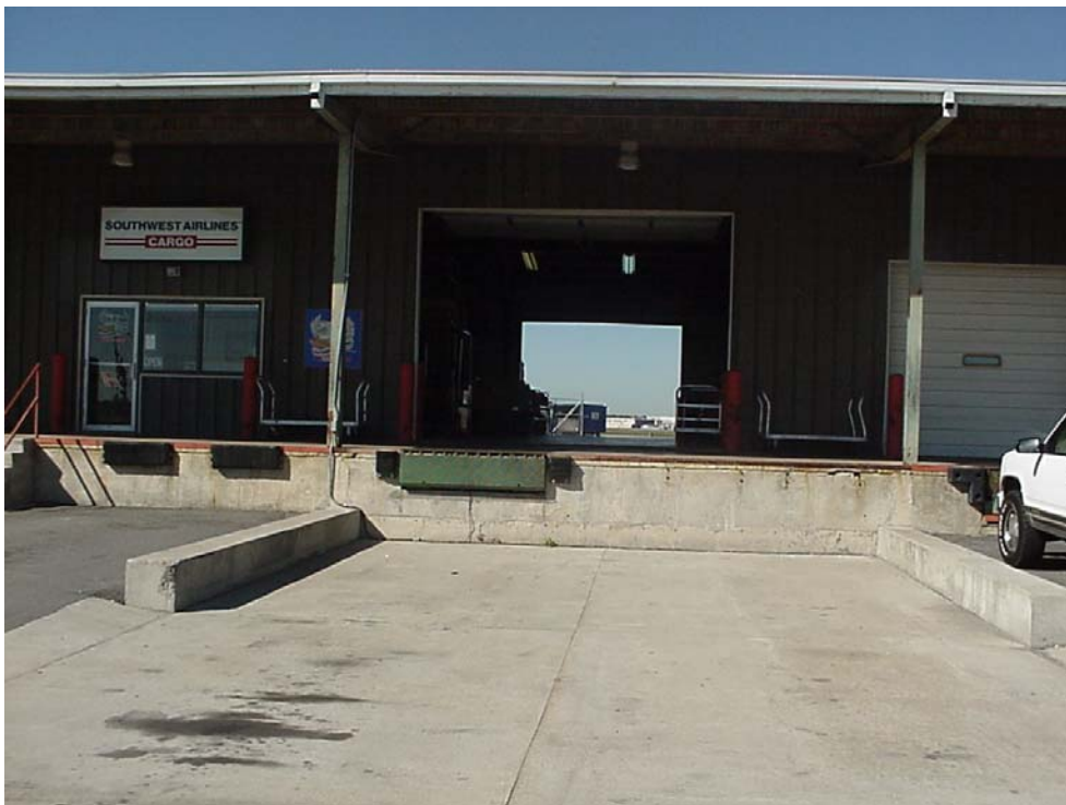
Southwest Airlines Cargo Building at Air Cargo Terminal
