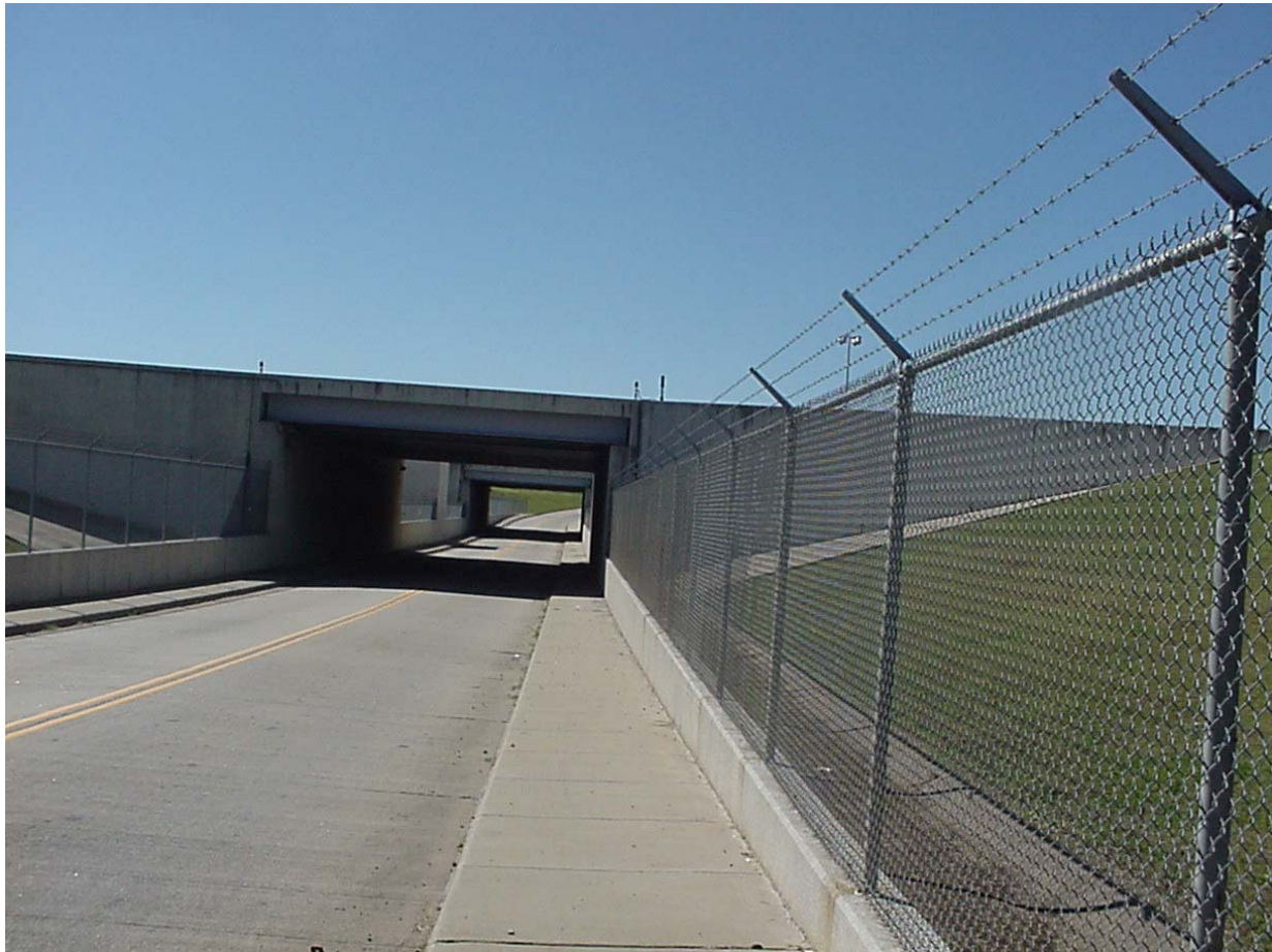
Taxiways over Temple Street
