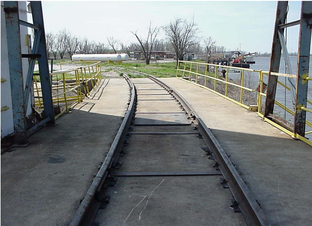
Railcar dumping station for conveyor transfers to barge
