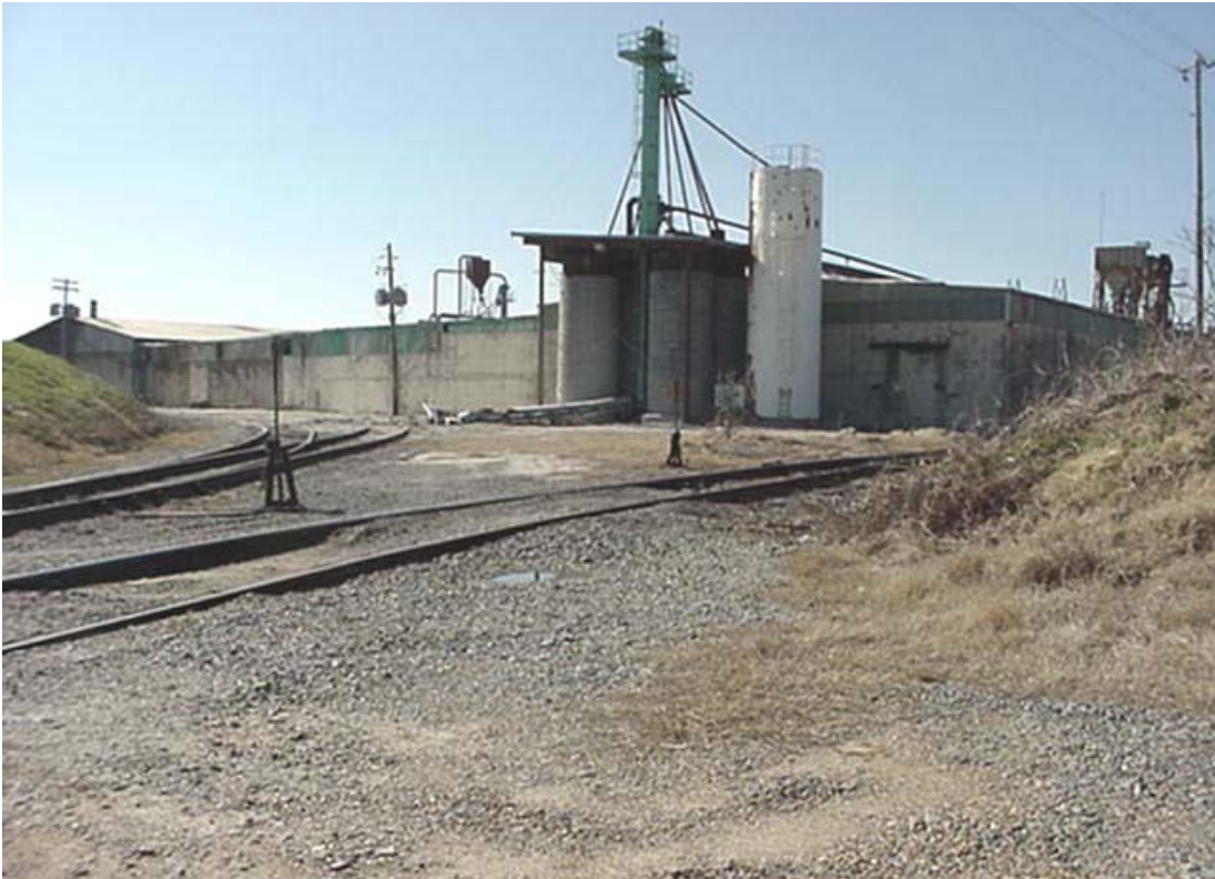
Rail entrance through the levee
