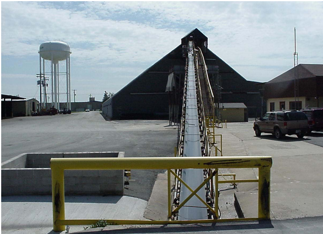
Chemical/fertilizer warehouse. Scale house shown on right
