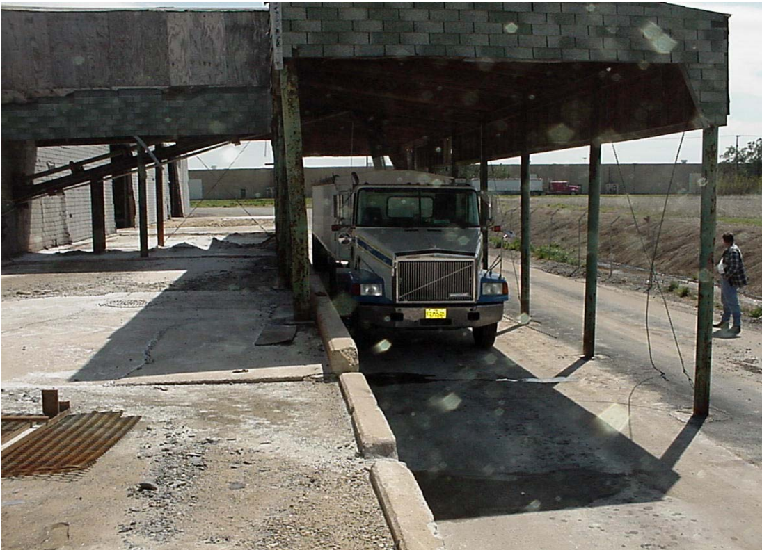
Interior conveyor transfers product to the covered loading dock
