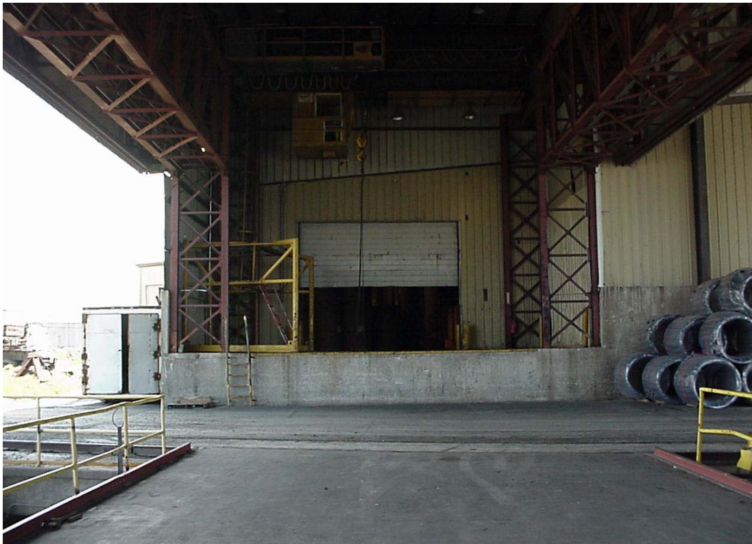
Covered overhead crane moves material from barge to train or warehouse
