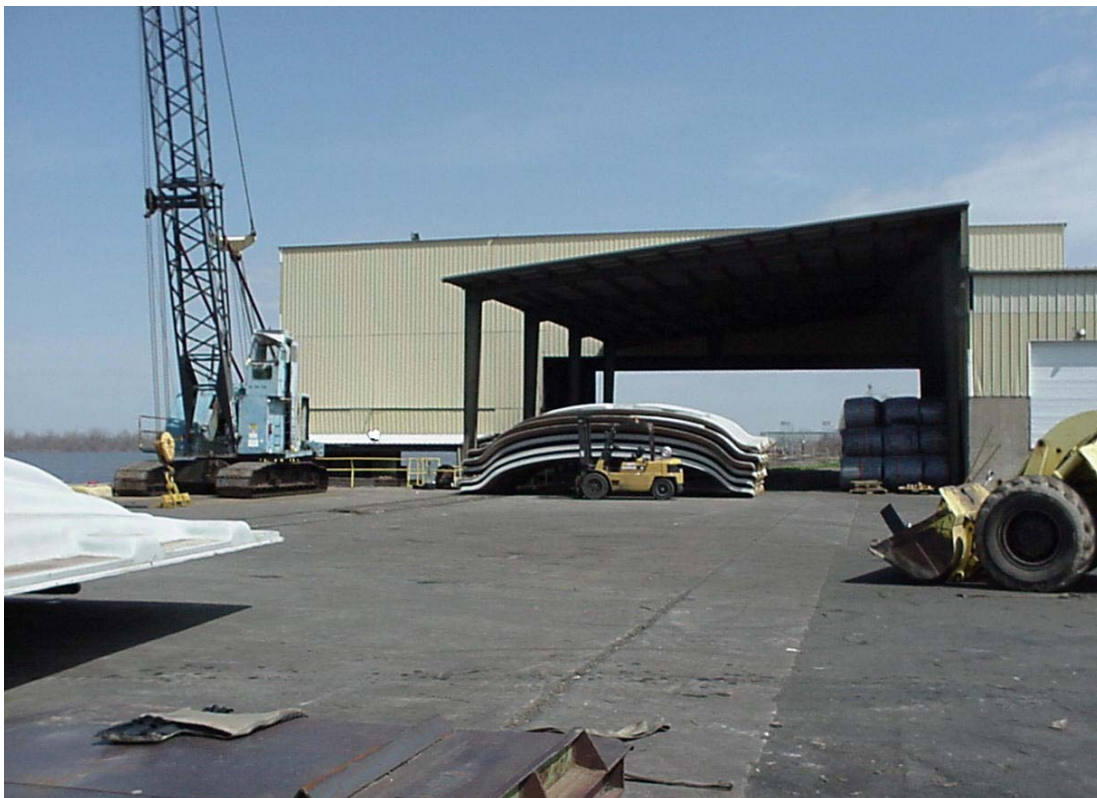
Full view of covered overhead crane area
