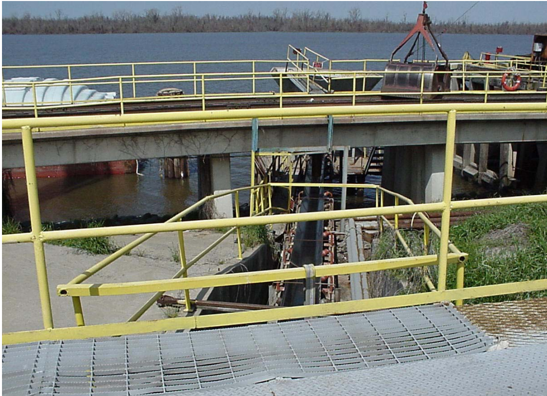
Conveyor used to offload barges
