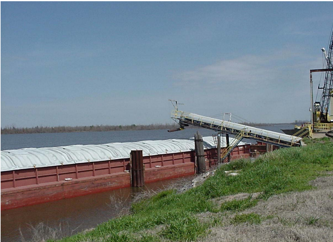
Conveyor for loading barges
