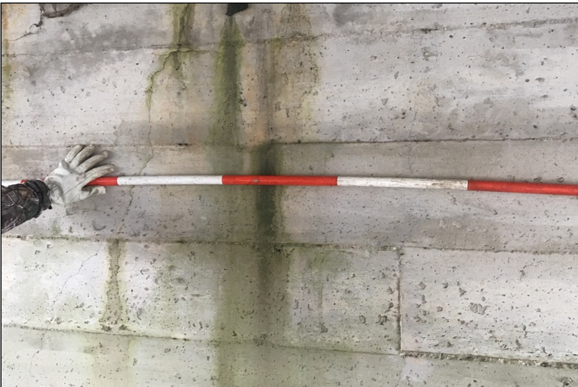
Bent 1 abutment has vertical cracks average width of 0.020".
