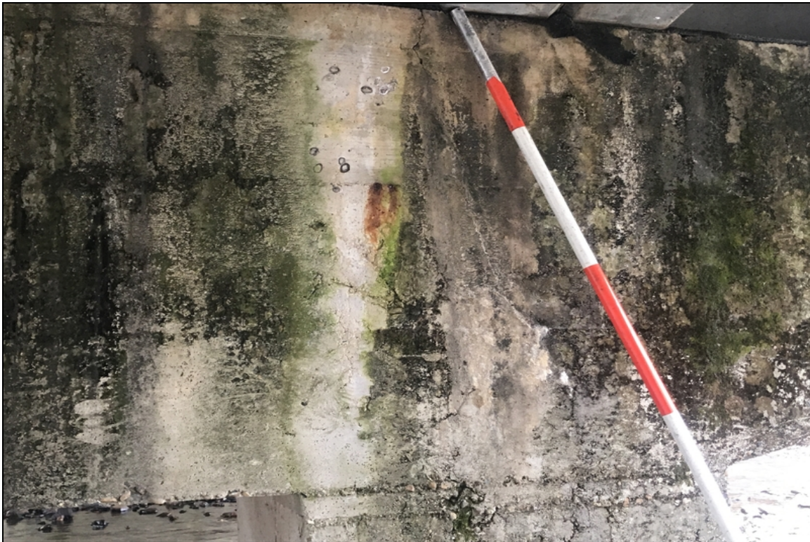
Bent 2 ahead column 1 has crack with efflorescence.
