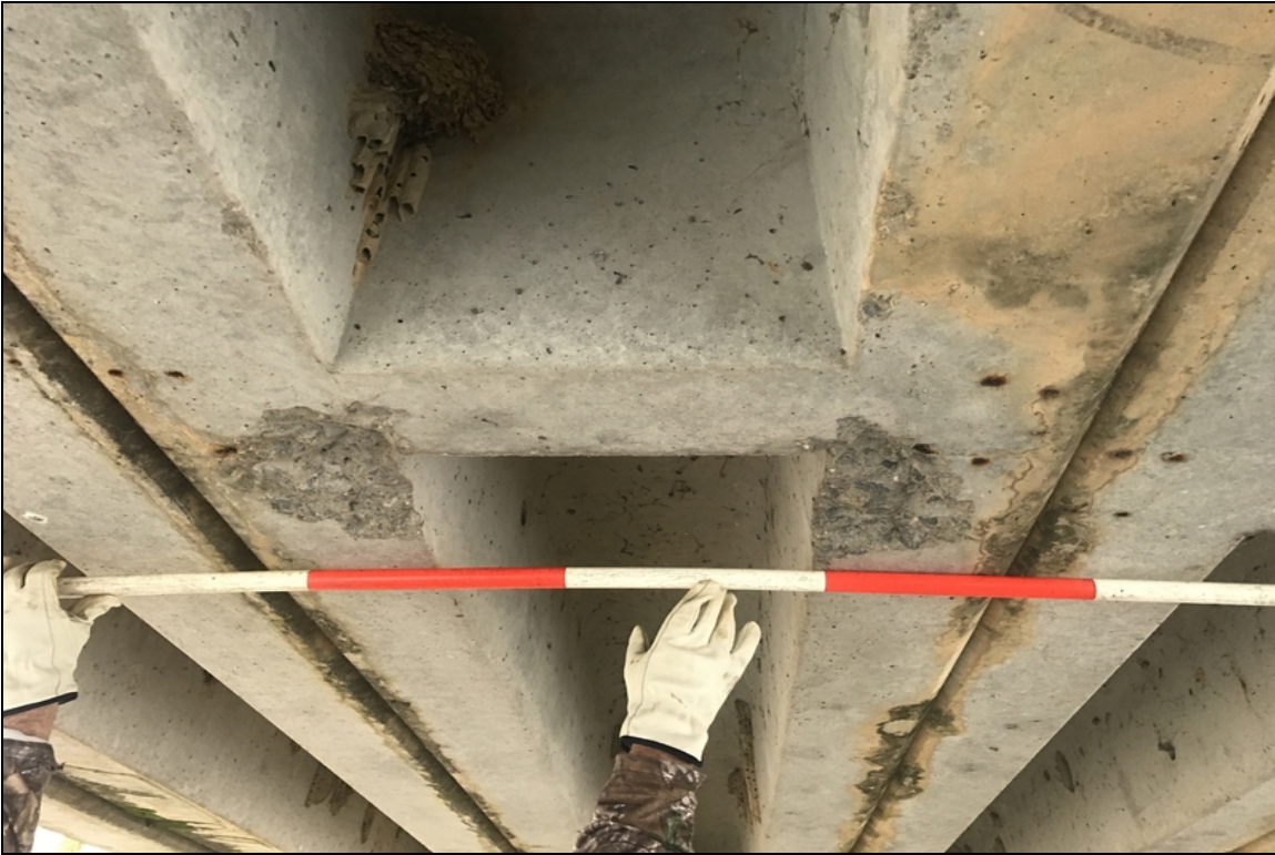
Span 1 channel unit 6 12' ahead of bent 1 has spalls in legs.
