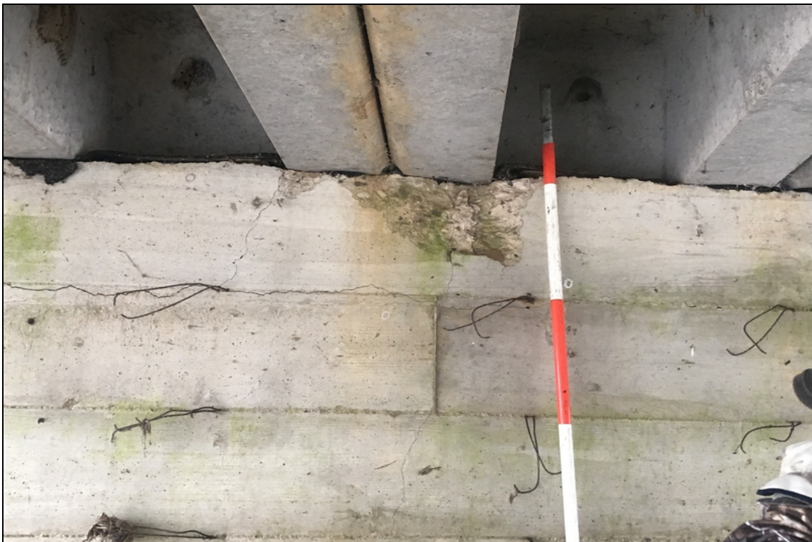
Bent 4 abutment has contact spall under channel unit 3.
