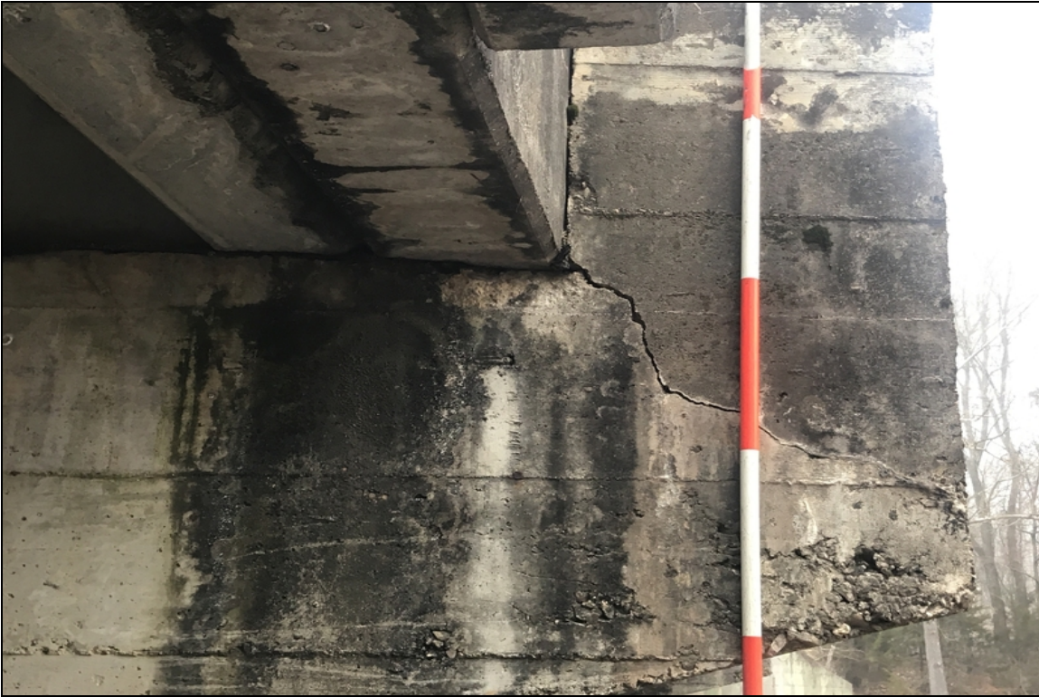
Bent 3 cap ahead face has crack and contact spall on right side.
