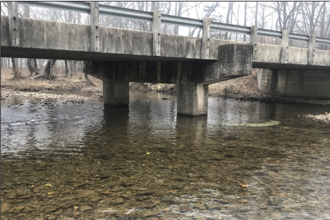
Logs wedged against bent 2 have been removed.
