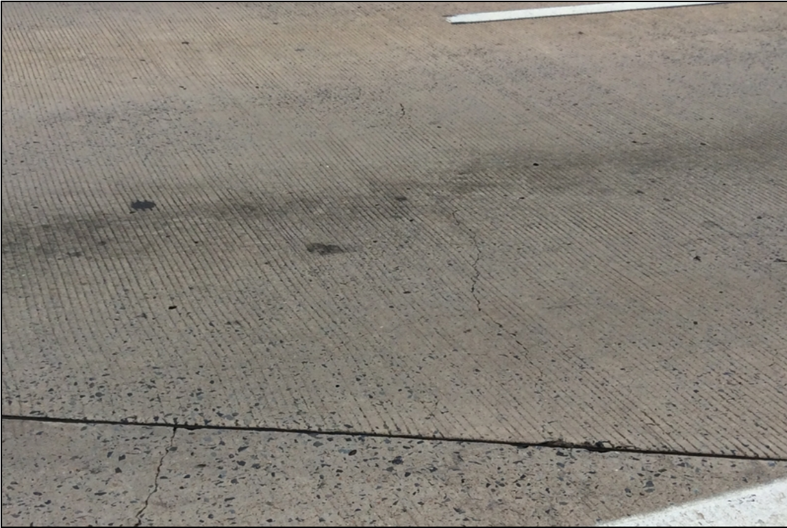
Deck at Bent 1 cracks up to 0.040"
