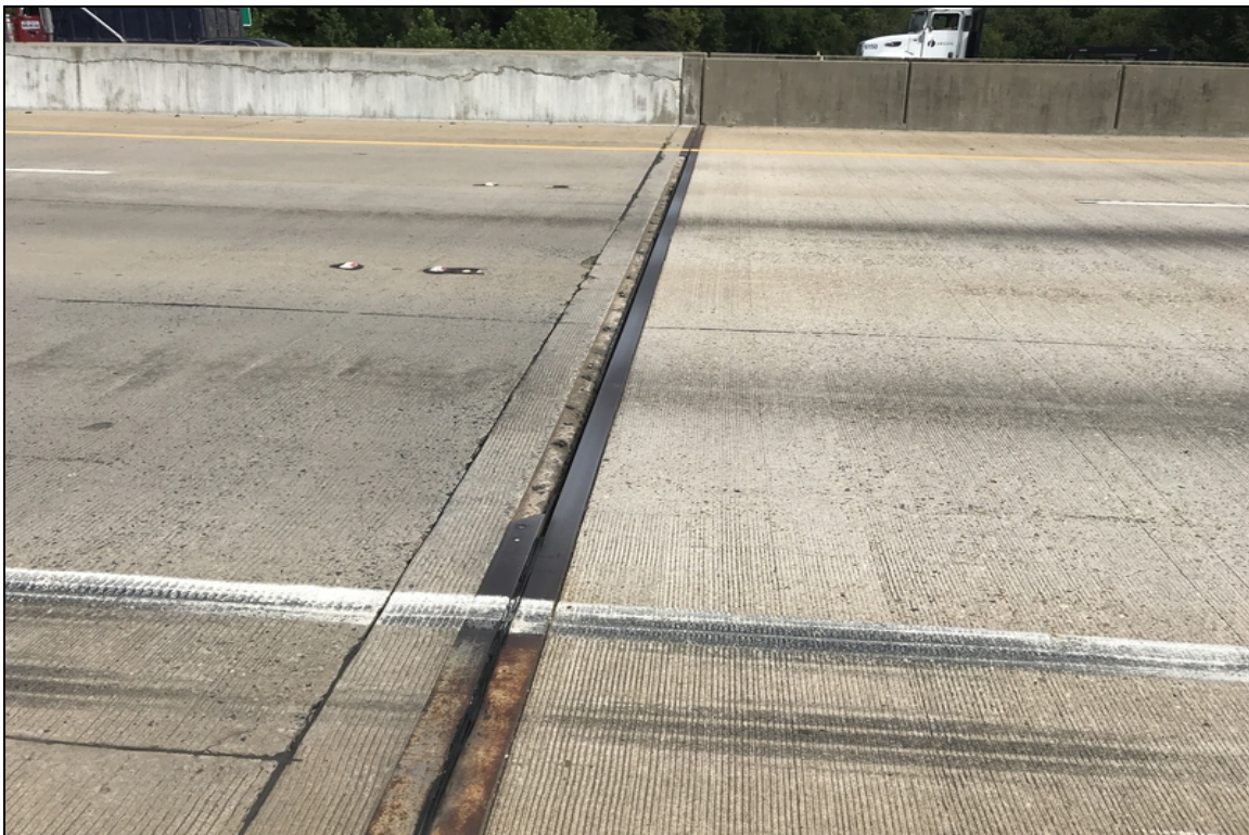
Bent 1 joint armor missing.
