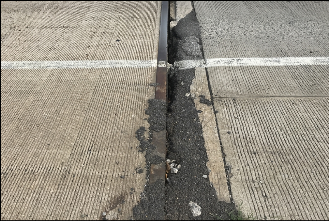
Bent 7 spall filled with asphalt in top of back wall
