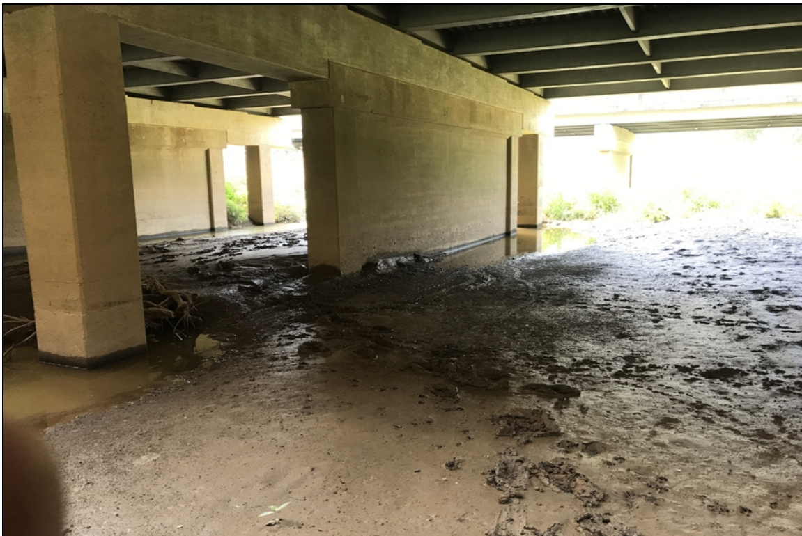
Bents 5 & 6 channel scour has been repaired.
