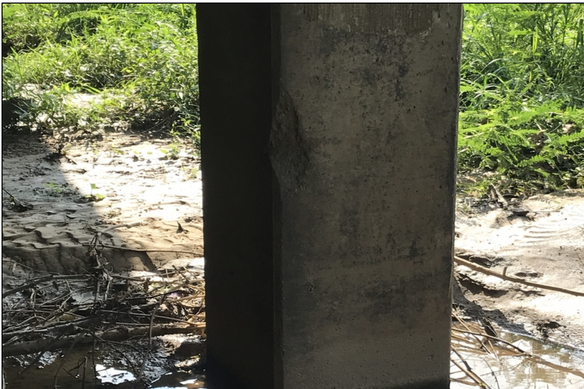
Bent 4 column 4 back spall
