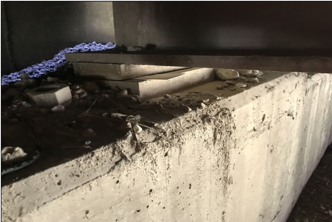
Bent 7 abutment, bearing at girder 5. Gap between bearing and masonry plate.
