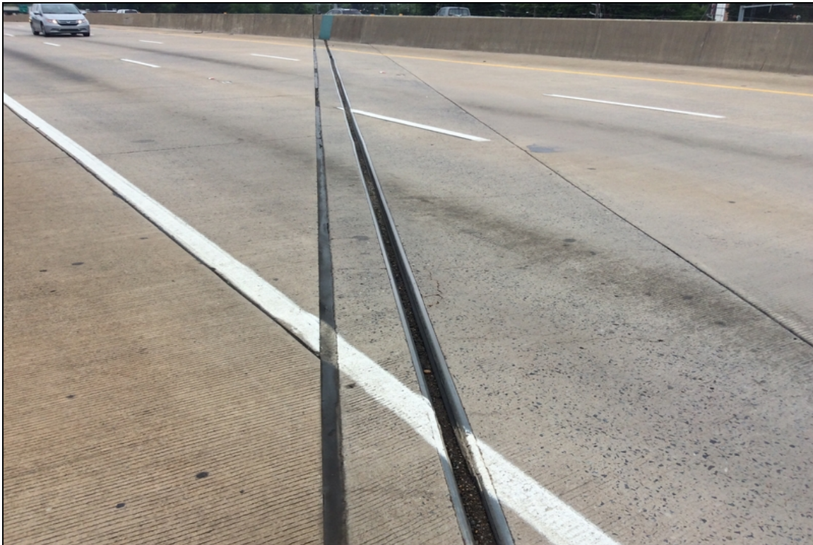
Bent 1 joint seal half full of debris
