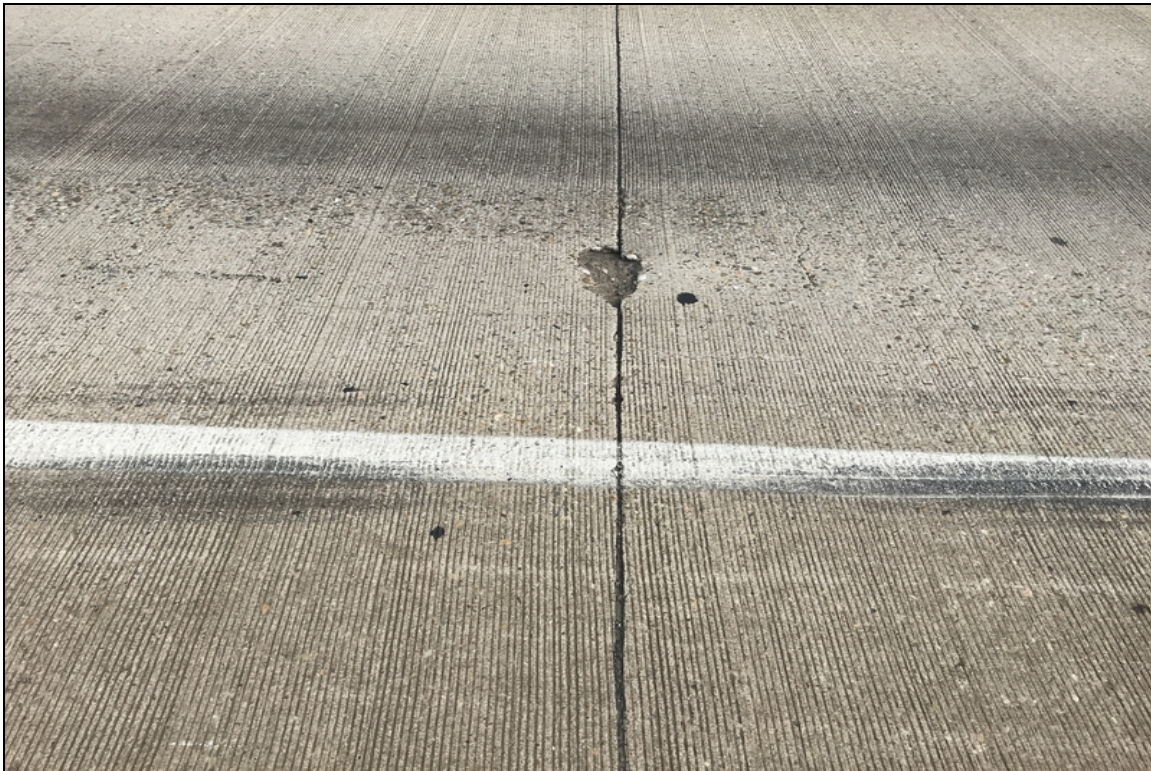
Deck bent 2 spall
