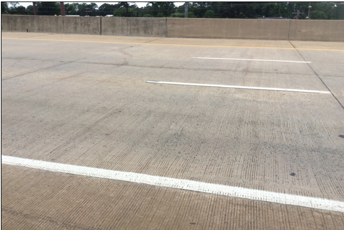
Large cracks in east approach slab.
