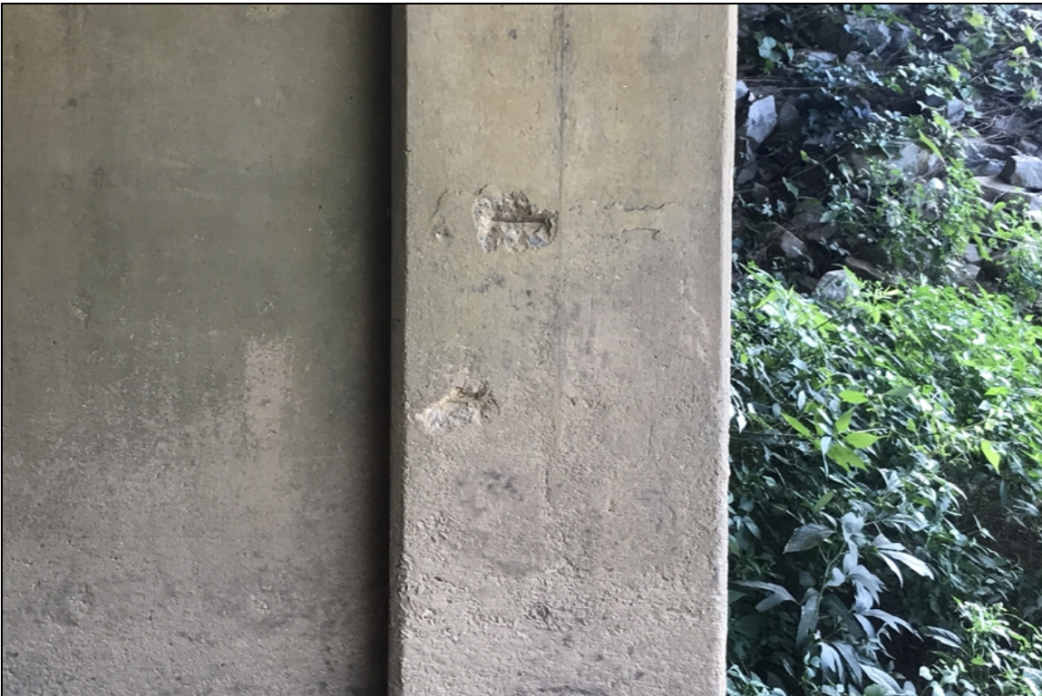
Bent 6 column back spall with exposed rebar.
