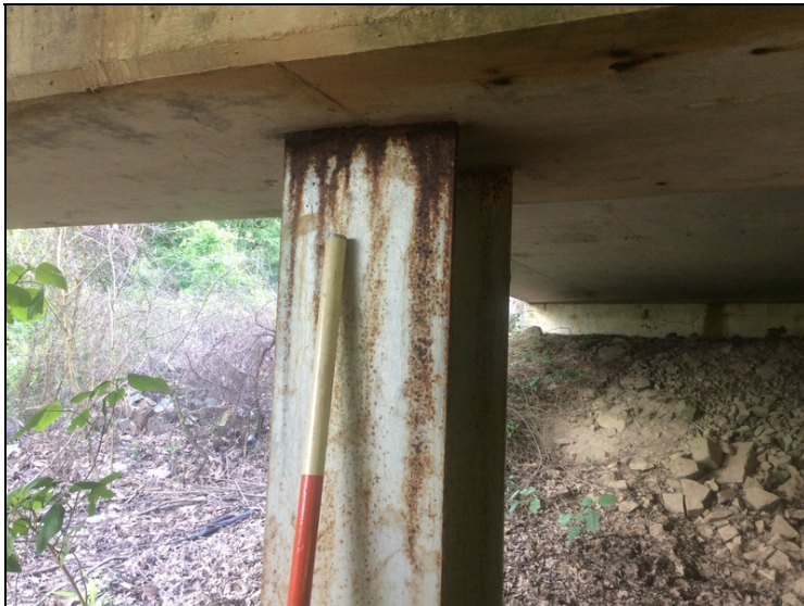
Steel pile 4 at bent 2 has moderate pitting at the top, common pile 2.
