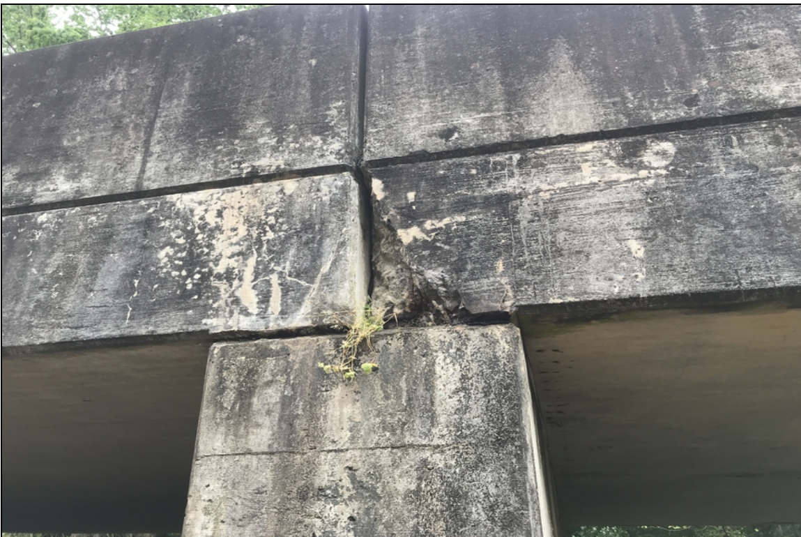
Span2 at bent 2 right side has spall with exposed rebar.
