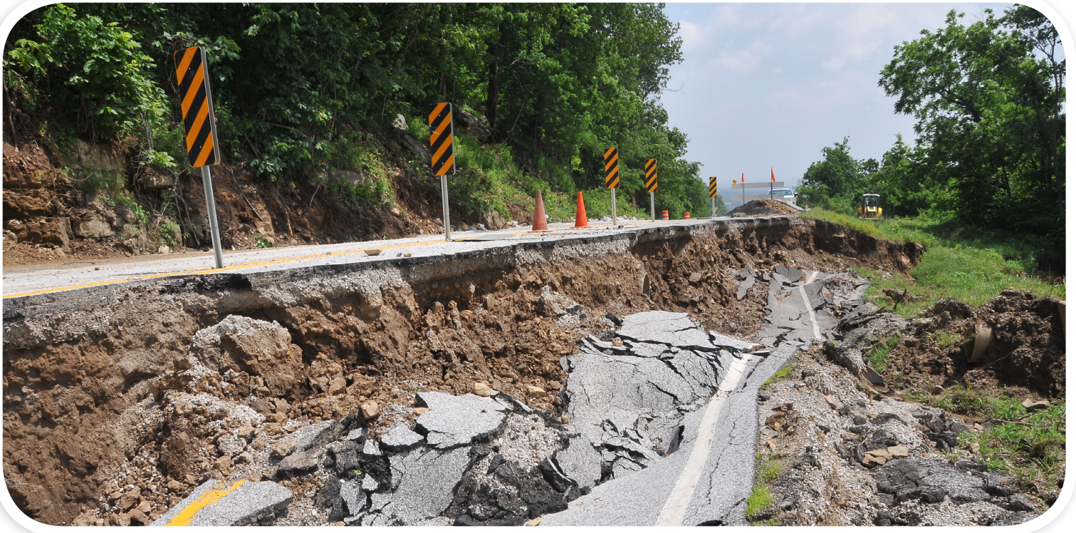
Highway 43 in Boone County
