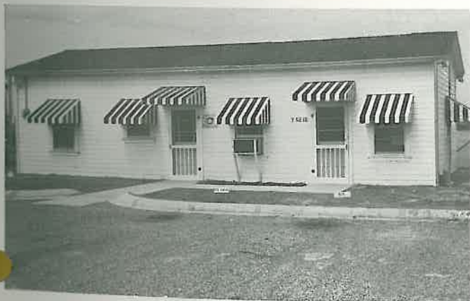
N. D. Pumphrey, resident engineer in District 7, calls this neat structure "home" when he is on the job. The building is in the area maintenance yard at Camden.
