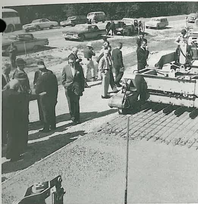
Inspecting the South Bypass
