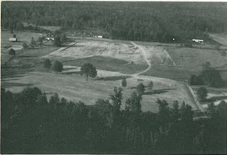
In the top picture is the progress being made on the District 10 headquarters building at Paragould; The bottom picture shows the land cleared for the new District 7 building at Camden.
