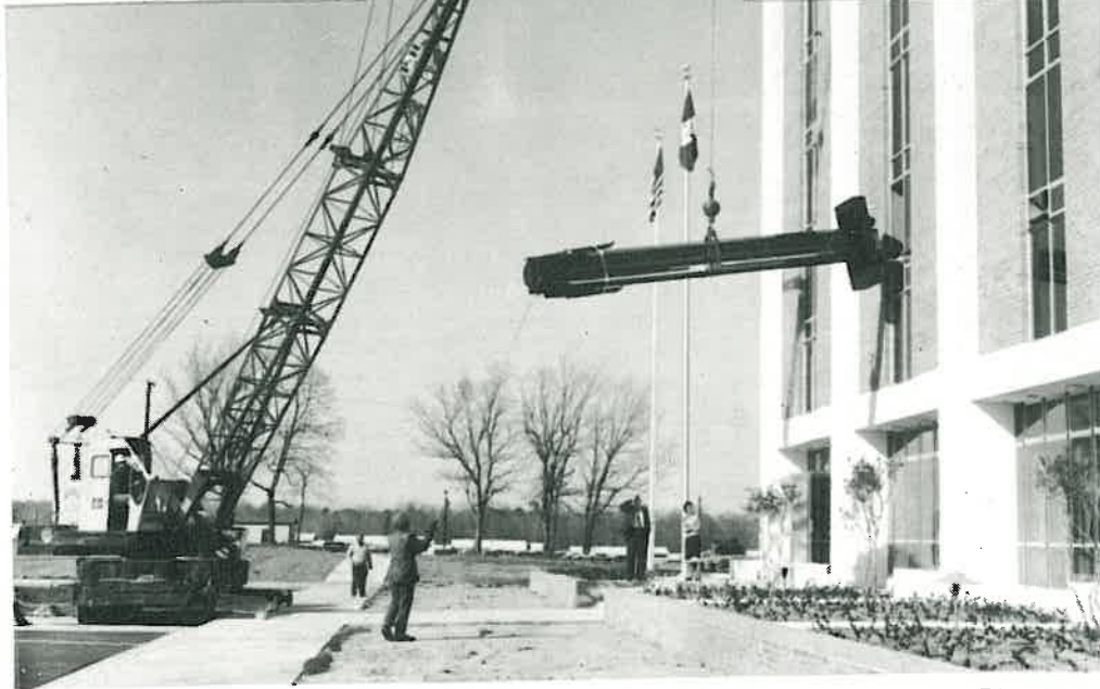
Delicate instruments to aid delicate instruments, though seemingly cumbersome. The crane is gently lifting the shaft of the new camera into the window.
