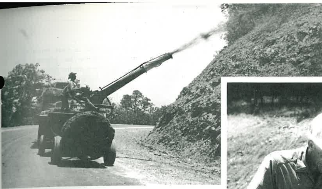
Seeding on the rugged slopes along Skyline Drive.
