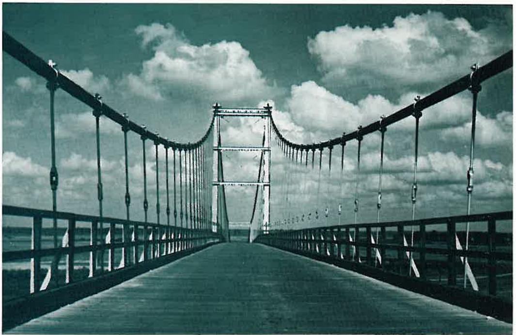
Modern traffic has long since outdated this narrow, wood-decked structure.
