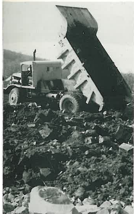
Rock from the ridge is used for fill elsewhere along the route. ←
