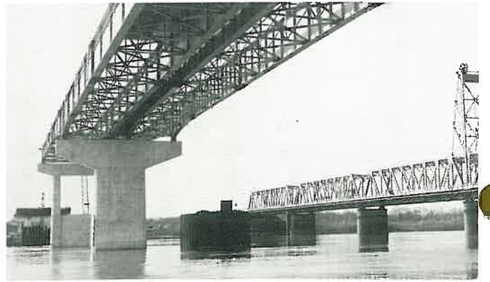
Looking toward Van Buren from under the new bridge.
