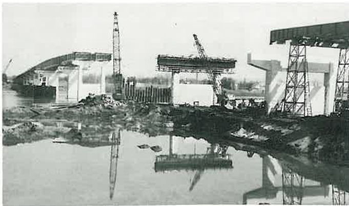
Pier construction of the Fort Smith-Van Buren bridge.
