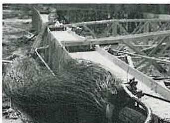
The explosive charge separated the hundreds of individual strands of the cable, giving it a hair-like appearance.
