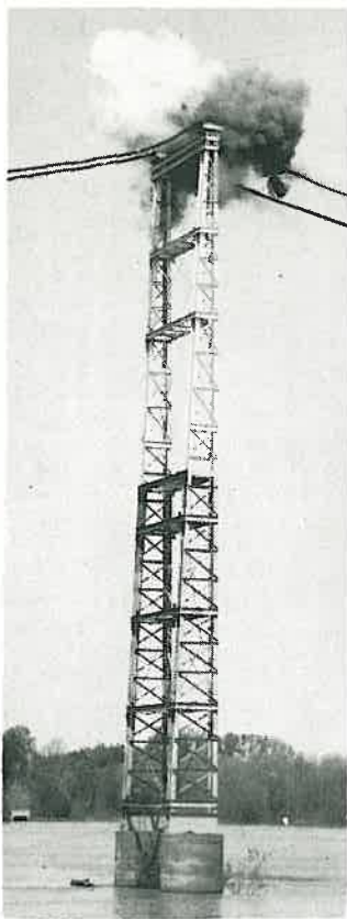
Demolition team member awaits signal to set off explosive which will bring down the bridge spans.
