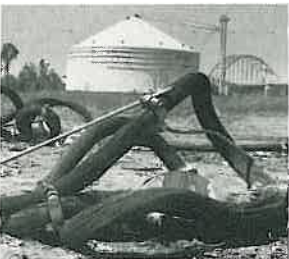
Massive cables which supported the bridge lay in a snarl after explosion brought them to the ground.
