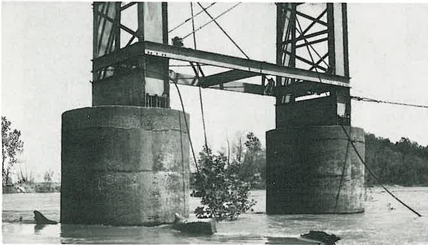
Bridge tower piers.
