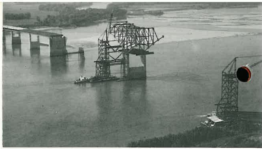
Steel being hung on the main channel superstructure.
