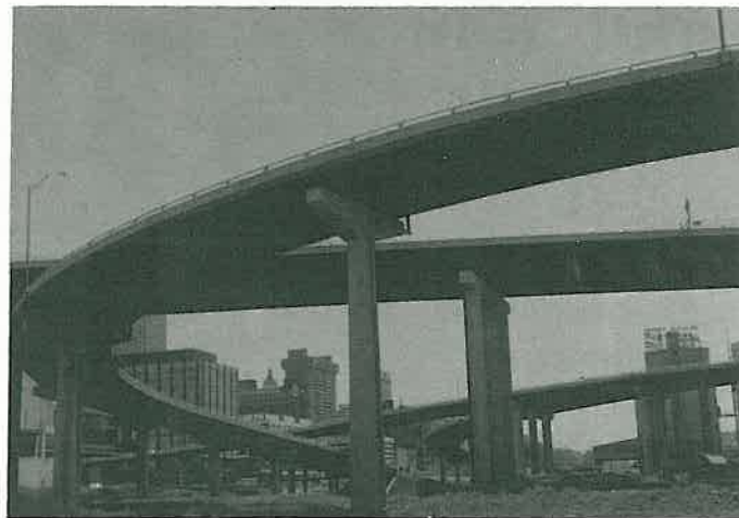
Bridge ramp on Memphis side.
