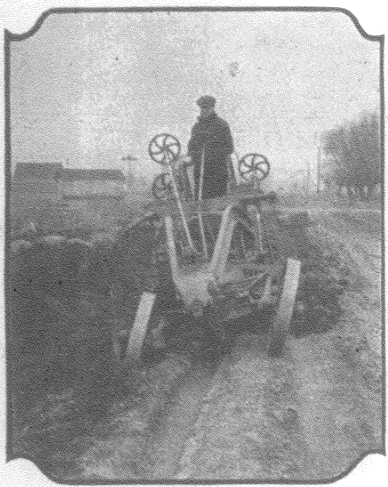
This Heavy Duty model, with Crawler Tread and steel-tired leaning front wheels, is working on a shoulder where a straight wheel machine could never be operated successfully.
