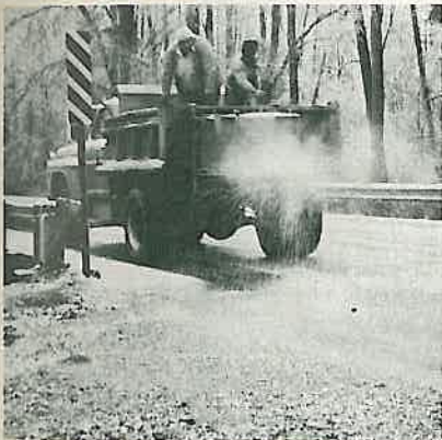
Two AHD employees put out sand on a bridge near Magnolia.
