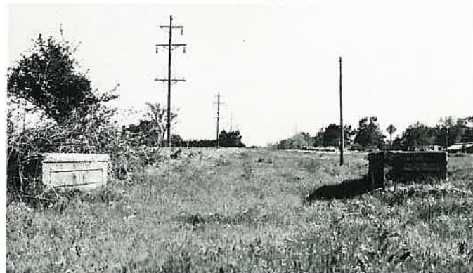
Last issue's Where Is It was the wing walls of an old bridge on a re-located section of Highway 1 near Caldwell School between Wynne and Forrest City. Billy Morgan of Hughes, a motor patrol operator, and Maint. Supt. C. W. George identified the picture.
