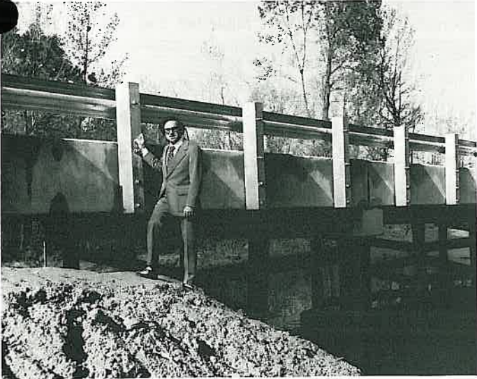
State-aid Engr. John Kizer stands beside the completed bridge near Smackover.
