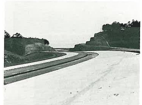
This hill doesn't look very steep, but just try it on a bicycle! Terraced cuts, as deep as 100 feet in some places, through formidable rock bluffs, were necessary to drop the highway 205 feet between Highway 10 and the river, slightly less than a mile away.
