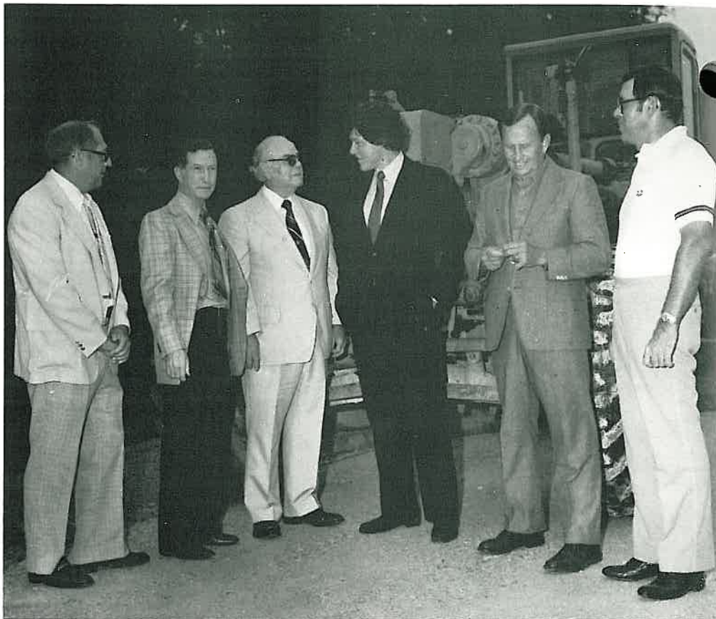
Inspecting work on Highway 65 at Harrison are: (left to right); Glen Feldman, President of the Harrison Chamber of Commerce; Jim Selby, Assistant District 9 Engineer; Hurley Perkins, District 9 Engineer; Governor Bill Clinton; Director Henry Gray; and Bill Bonsteel, Chairman of the Harrison Chamber Commerce Transportation Committee.
