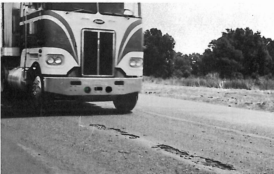
The asphalt pavements across the state took a beating from the extreme heat and heavy truck traffic.
