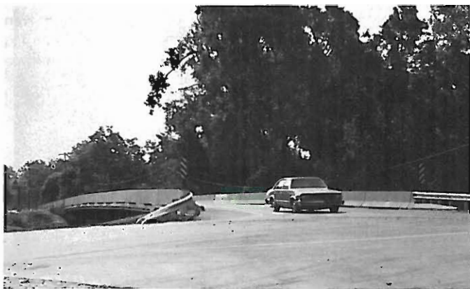
Bridge over Fourche Creek in Pulaski County.
