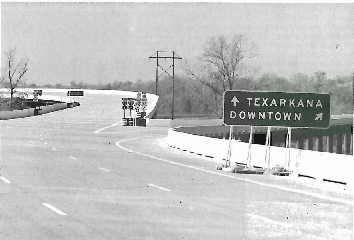
South terminal interchange looking west
