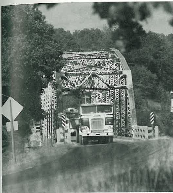
The Fourche LaFave River Bridge on Highway 71 is one of three narrow structures the Department plans to replace.
