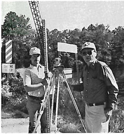
Leonard Johnson, left, an employee of four years, and Frank Novak, with 28 years of service, are working on the construction crew at the site of the new Saline River Bridge on Highway 160.
