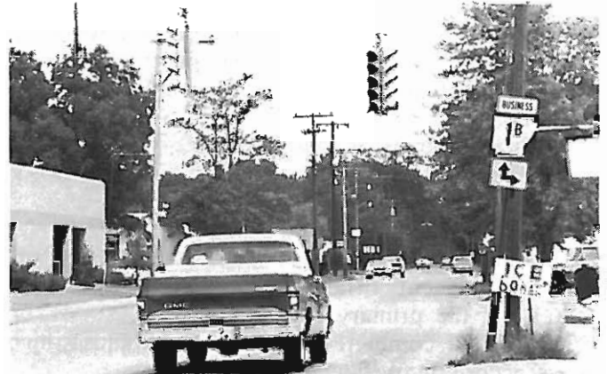
Highway 1B in DeWitt
