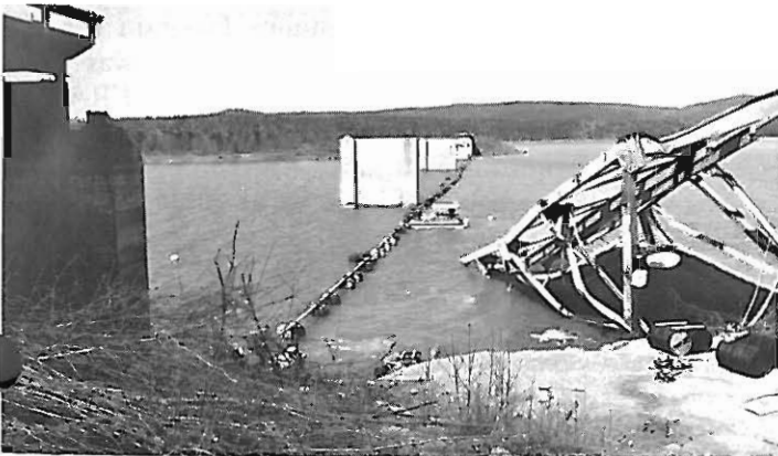
(Left to Right) The steel truss is seen laying next to the piers following the 1984 tornado. . . After modifying the piers, workers begin to hang steel for the new bridge.
