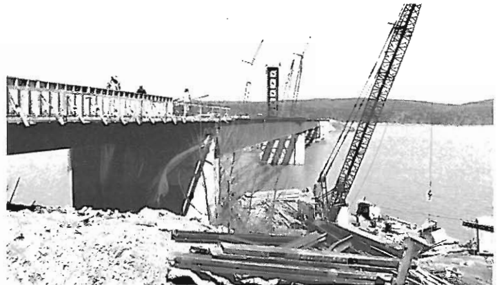
(Left to Right) The steel truss is seen laying next to the piers following the 1984 tornado. . . After modifying the piers, workers begin to hang steel for the new bridge.
