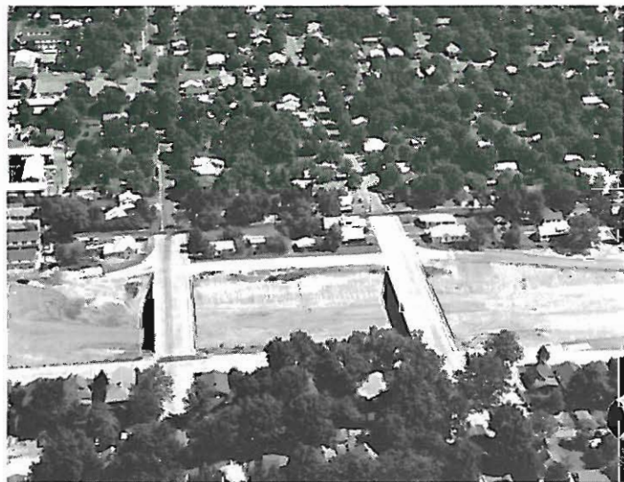
The Cedar/Pine Interchange on I-630 in July 1968.
