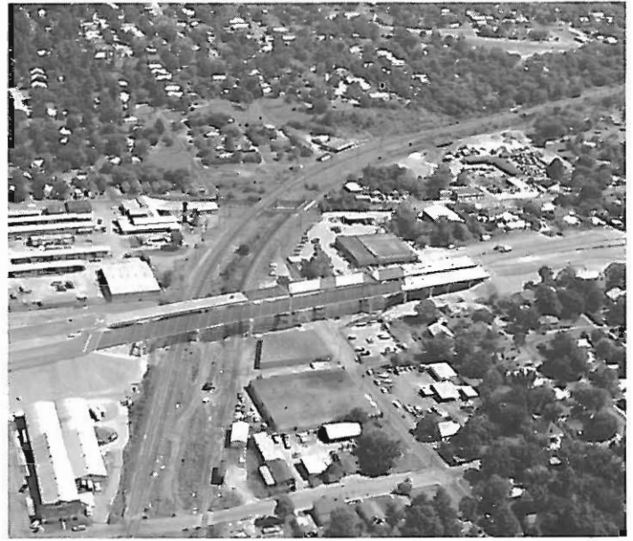
I-630 Railroad Overpass east of Woodrow Street, July 1968.
