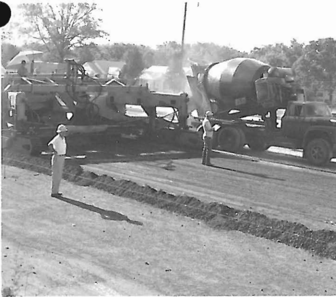
Paving on the first section of I-630 in August 1968.
