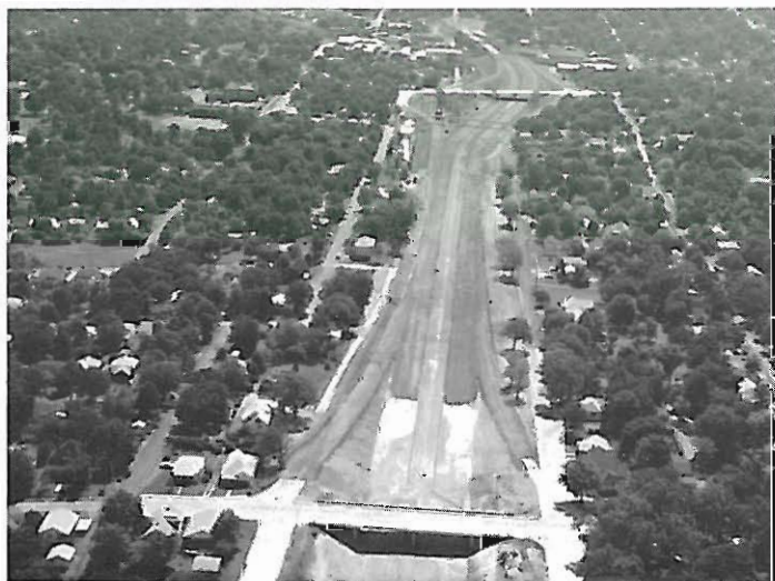
I-630 under construction looking east from the Cedar/Pine Interchange, July 1968.
