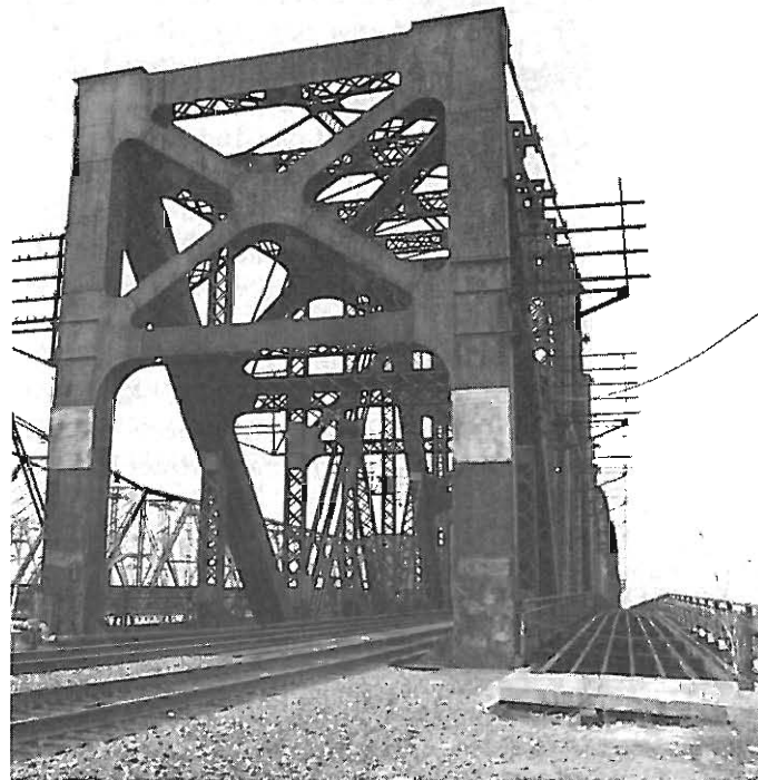
The Harahan Bridge was built in 1916. Wagons, and later, automobiles, used the outside deck as a means of crossing the river. The wooden deck has since been removed but the supports which remain can be seen to the right.
