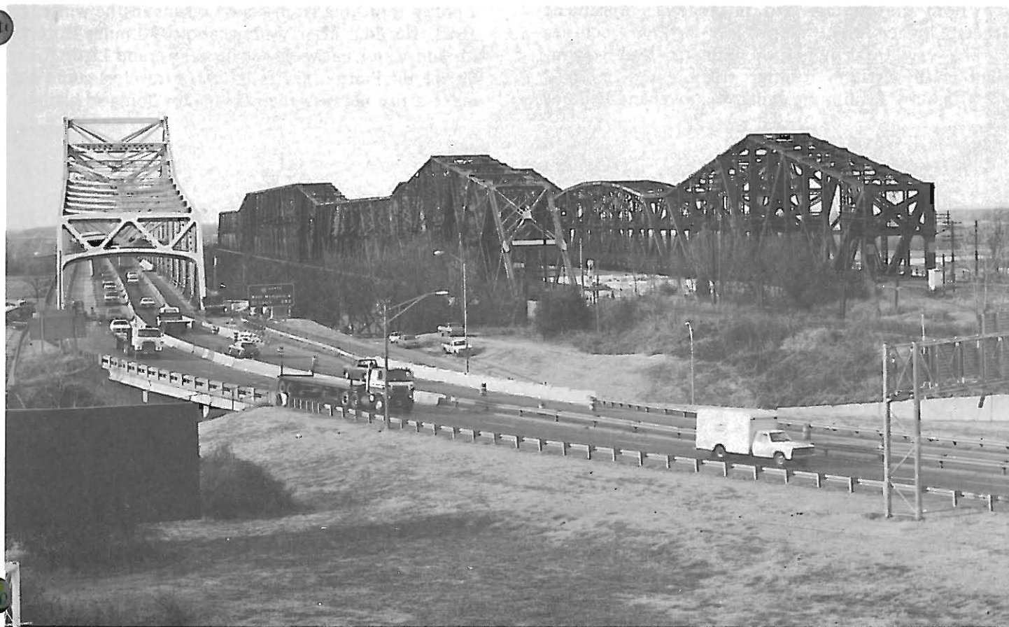
The I-55 Bridge, to the left, is presently undergoing major rehabilitation work. The center bridge is the first one built across the Mississippi River at Memphis and the bridge to the right is the Harahan Bridge.
