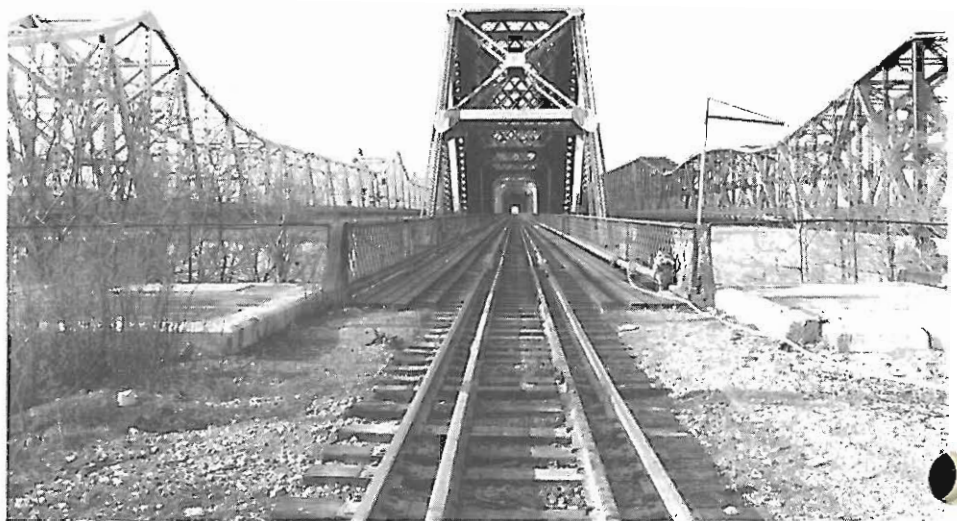
The first bridge over the lower Mississippi River was completed in the early 1890's. The single-track railroad structure also served as a pedestrian and wagon crossing.
