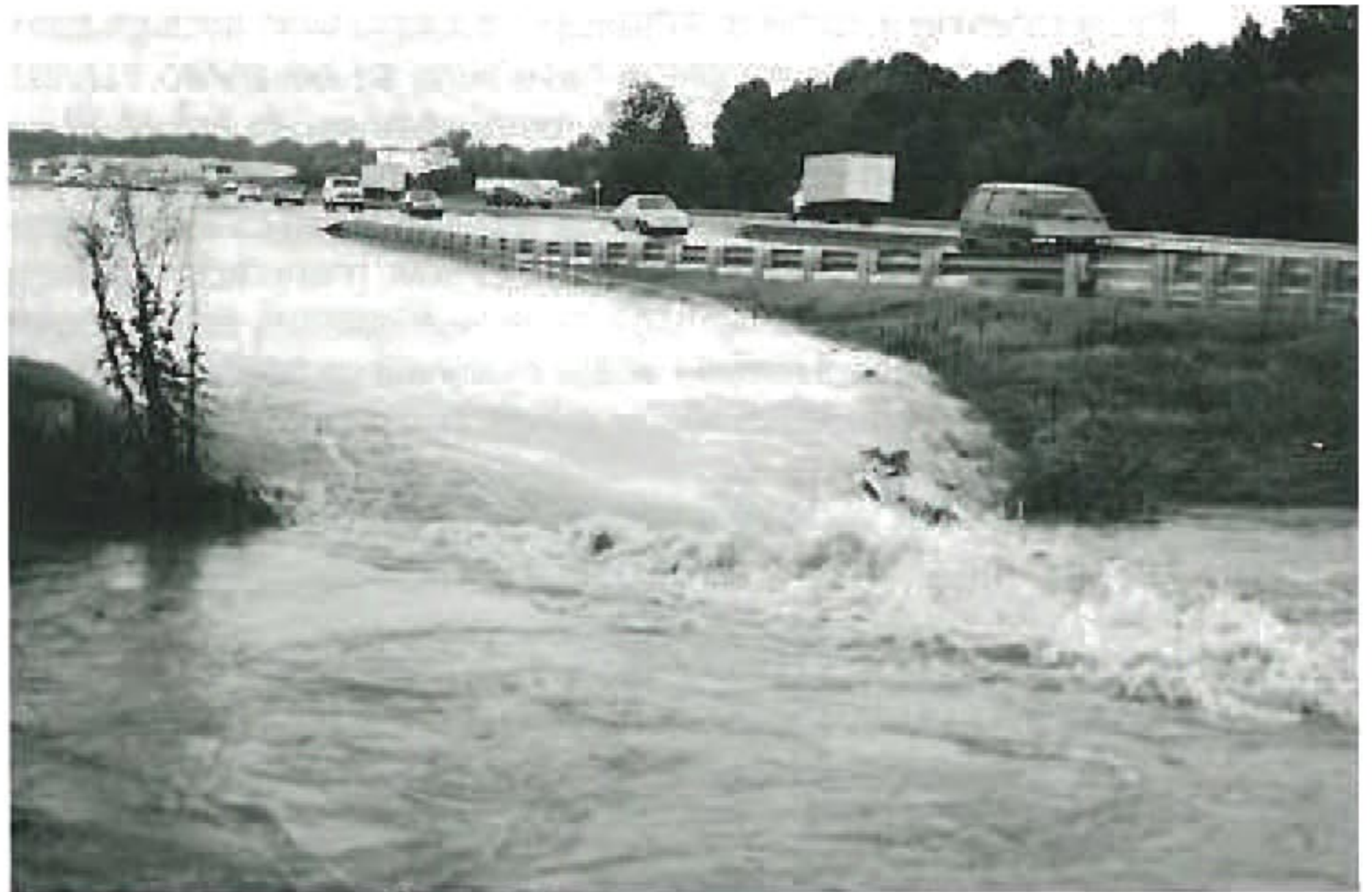
Flash flooding throughout Arkansas created numerous problems for department personnel.
