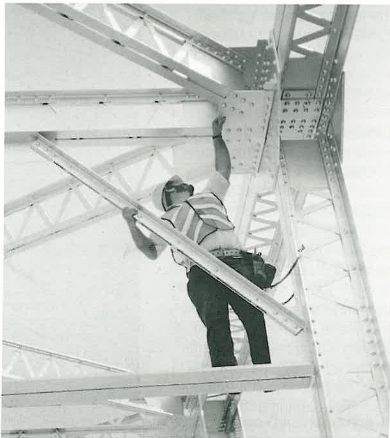
The inspection of steel members.
