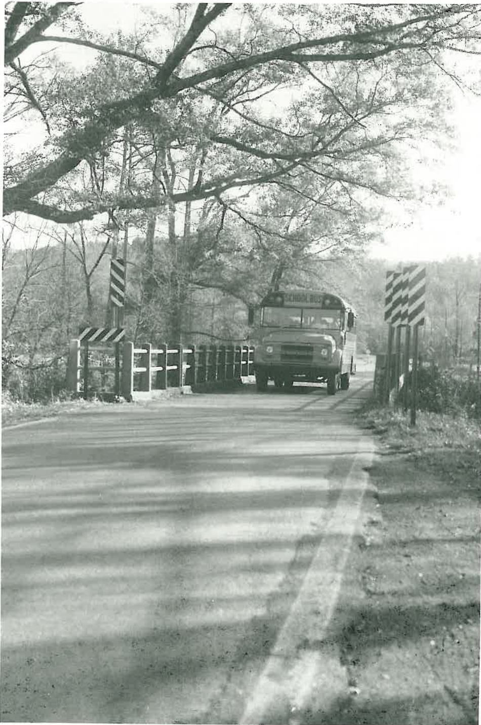
A typical example of a narrow, one-lane functionally obsolete bridge in Arkansas.
