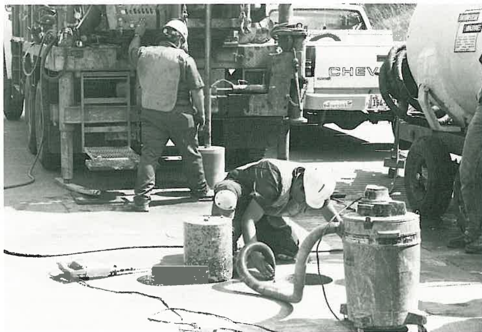
Workers remove concrete core samples from Interstate 430.
