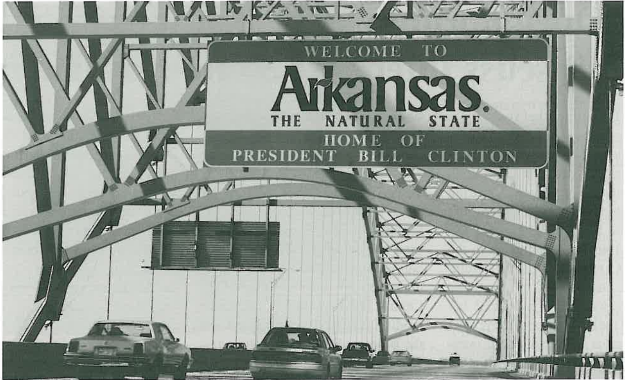
The new "Welcome To Arkansas" sign on the Interstate 40 Bridge at West Memphis
