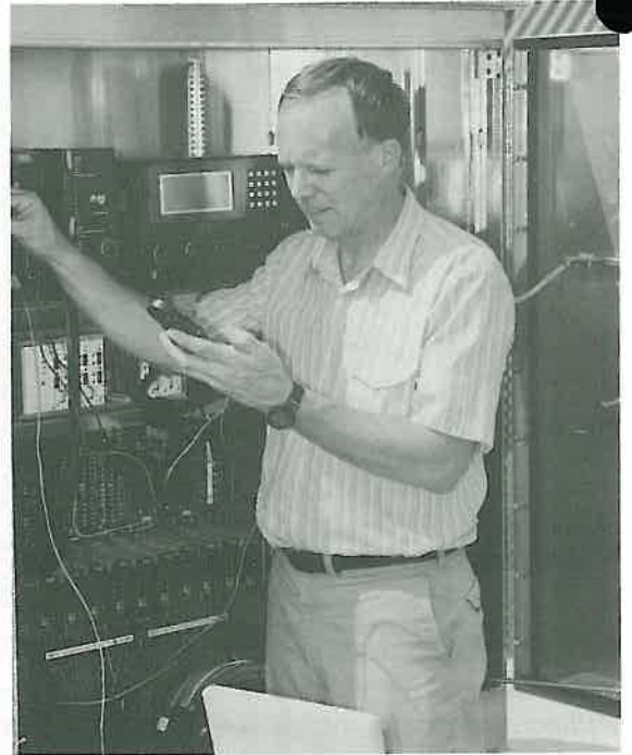
Mark Lyons , Senior Traffic Engineer for Roadway Design, calibrates a main signal box on State Highway 49 in the city of Helena.
