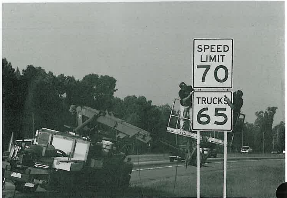
On August 19, AHTD sign crews installed 70 m.p.h. signs.
