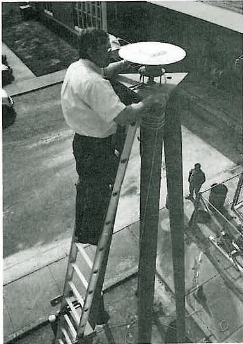
Mike White, Staff Surveys Engineer, attaches a monitor cable to a CORS tower.
