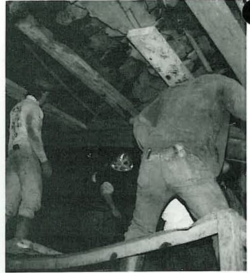
Employees of J.F. Shea Co. help place the final support structures.
