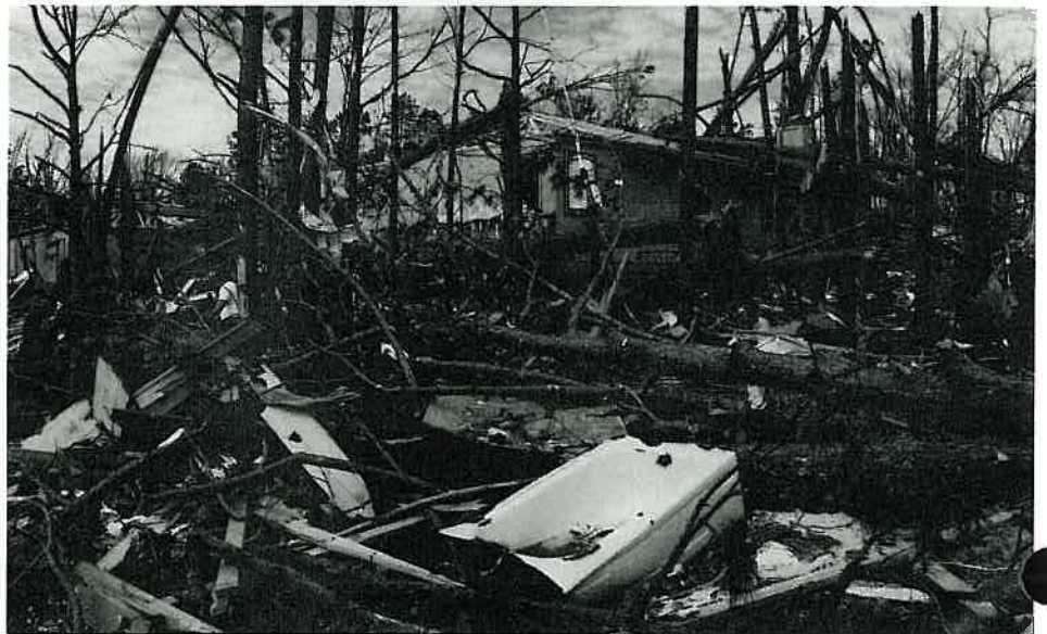
All that remains of Carlotta Vaughn's home on Blueberry Drive in Southwest Little Rock
