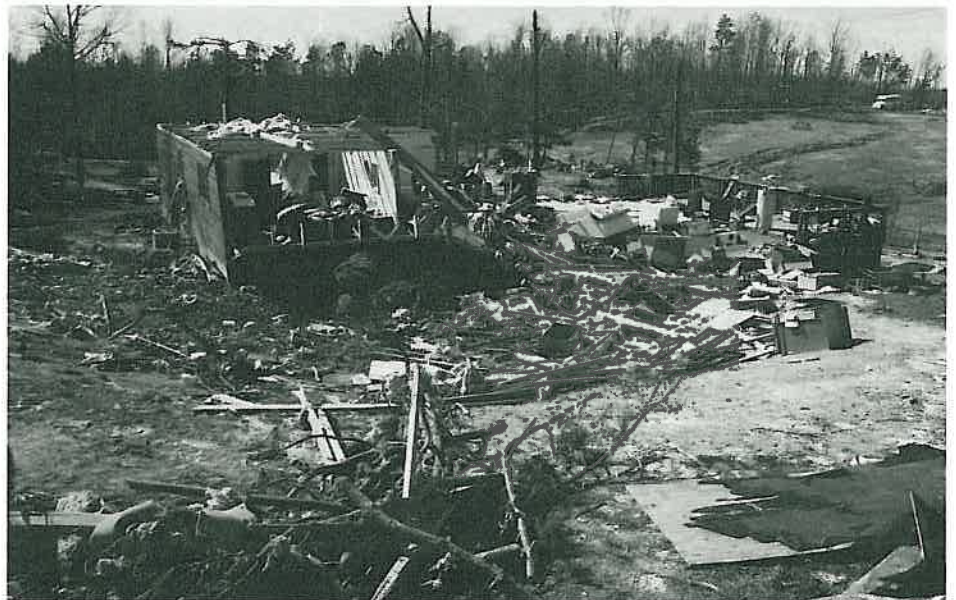
The remains of Danny Moore's home after the March 1 tornado. Moore plans to rebuild on this site.
