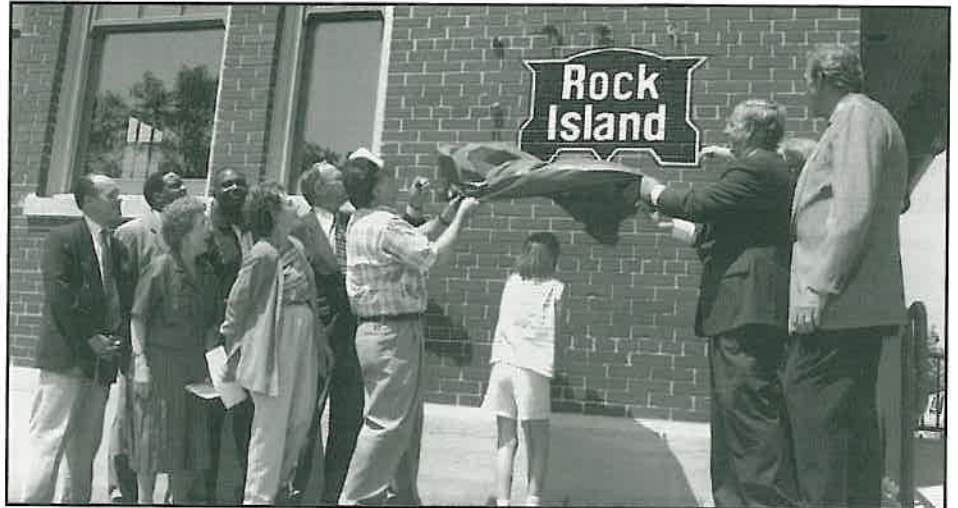
North Little Rock Mayor Patrick Hays, left, and AHTD Director Dan Flowers, right, unveil the Rock Island emblem on the side of the restored depot.
