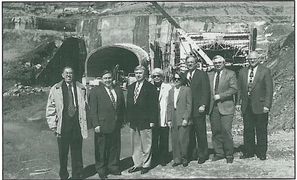
Standing in front of the entrance to the Bobby Hopper Tunnel are Chairman Bobby Hopper, Vice Chairman Herby Branscum, Jr., Commissioner John Lipton, AHTD Chief of Administration and Public Affairs Jane Wilson, Commissioner Prissy Hickerson, AHTD Director Dan Flowers, AHTD District 4 Engineer Harold Beaver, and AHTD Deputy Director and Chief Engineer Roger Almond.
